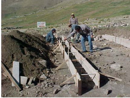
Figure 13: Plain concrete foundation
