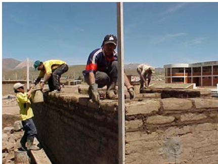
Fig. 27: For new houses, check the width of joints and use connector wires in the joint
