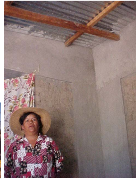
Figure 15: Interior wall strips and roof wood beams
