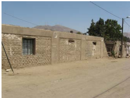
Fig. 19: House in Ica after the 2007 earthquake, reinforced walls undamaged.
