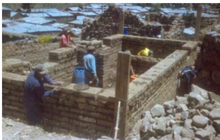
Fig. 30: Adobe walls under construction
