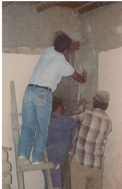
Fig. 25: Placement of vertical strip of mesh at a corner
