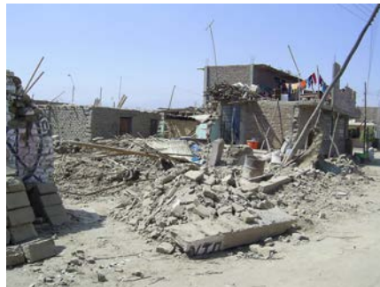
Fig. 23: Houses next to the one shown in Fig. 22, with heavy damage, Ica, 2007.
