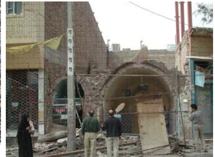
Figure 14: If walls can be kept in-plane, building typically survives. Adobe house in Bam earthquake.
