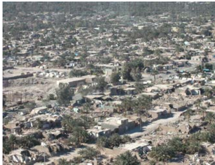
Figure 13: Aerial view of neighborhood with widespread damage to adobe structures in Bam earthquake
