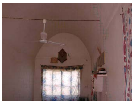
Figure 18: Basic gravity strengthening technique used for several hundred years--iron rod across vaulted space, tying walls together (increases gravity resistance, not seismic resistance)
