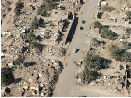
Figure 12: Aerial view of complete destruction of adobe dwellings in Bam earthquake
