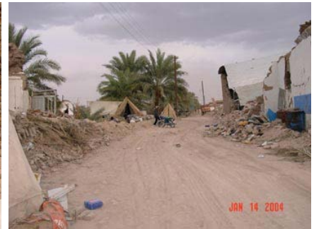
Figure 17: Bam earthquake: debris cleared from roadway, partially collapsed adobe structures, tents
