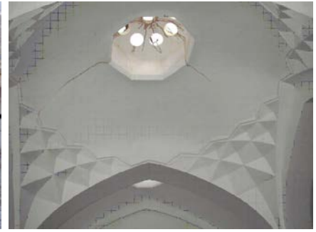
Figure 6: Ceiling skylight in wealthy adobe dwelling
