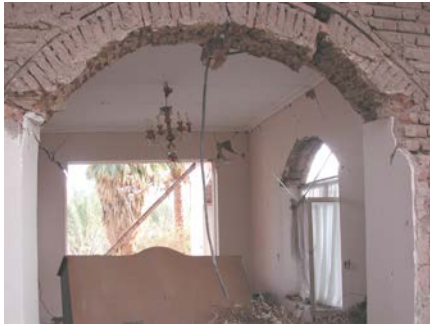
Figure 15: Bam earthquake: Damage to a traditional adobe house. Nonbearing walls collapsed, bearing walls are still standing.
