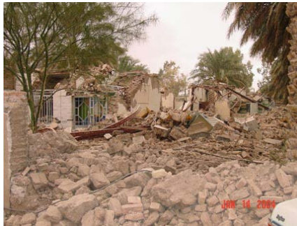
Figure 16: Bam earthquake: collapsed adobe structures
