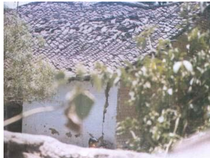
Figure 9b: Corner Separation
