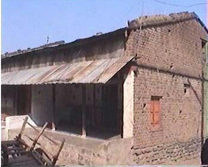
Figure 1b: Typical Brick Building With Timber Frame
