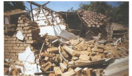
Figure 10: Damage to partition wall
