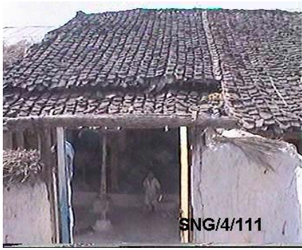
Figure 13: Heavy Roofing Elements
