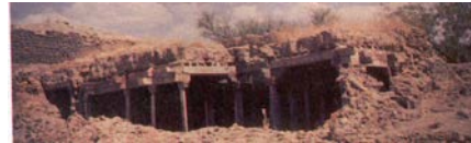
Figure 7: Damage Pattern of Building
