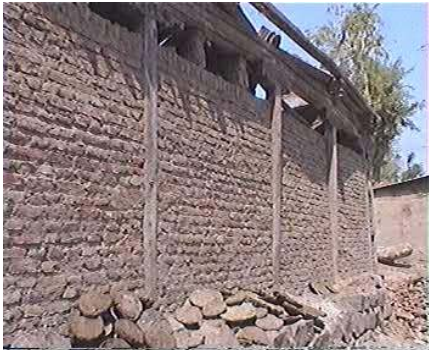
Figure 4a: Details of Timber Frame
