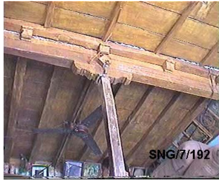
Figure 5a: Column and Beam Joint
