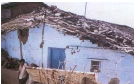
Figure 11a: Gable Failure
