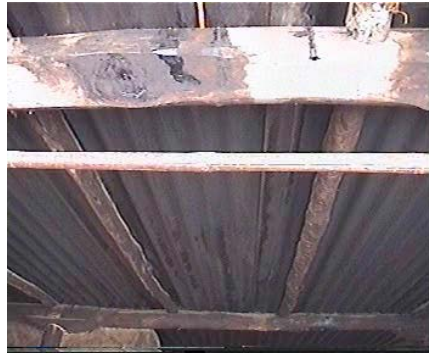
Figure 14: No Proper Joints Between Rafters and Purlins
