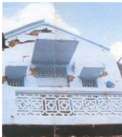
Figure 11b: Gable Failure
