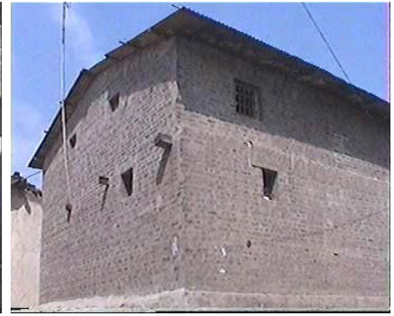
Figure 15: Houses Are Covered With Galvanized Iron Sheet
