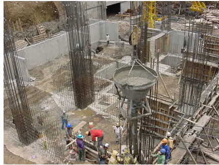
Figure 8: Construction view, Santa Fe Building
