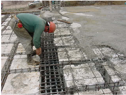
Figure 7: Floor construction, Santa Fe Building
