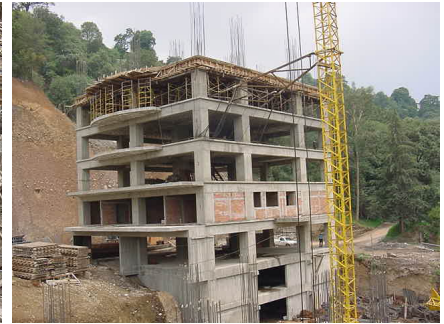
Figure 9: Santa Fe Building during construction
