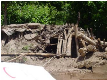
Figure 26b: Typical roof damage in Firoozabad-Kagoor earthquakes [3]
