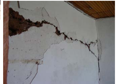
Figure 24a: Typical internal walls damage in Firoozabad-Kagoor earthquakes [3]
