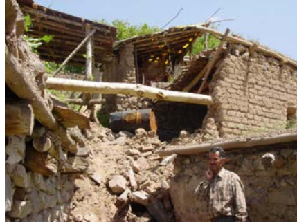
Figure 25: Typical roof damage in Firoozabad-Kagoor earthquakes [3]
