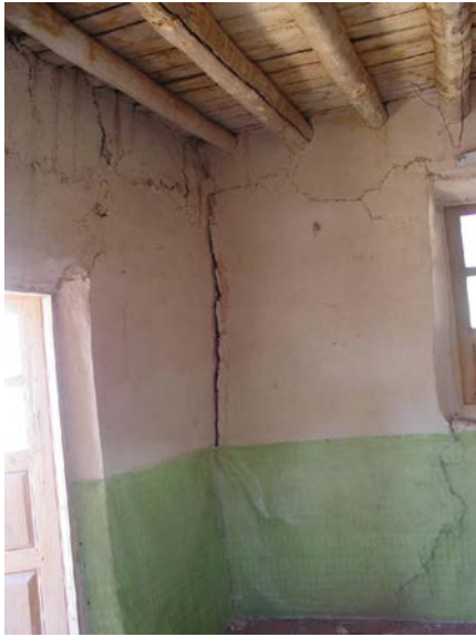
Figure 24b: Typical internal walls damage in Firoozabad-Kagoor earthquakes [3]
