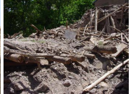
Figure 26a: Typical roof damage in Firoozabad-Kagoor earthquakes [3]
