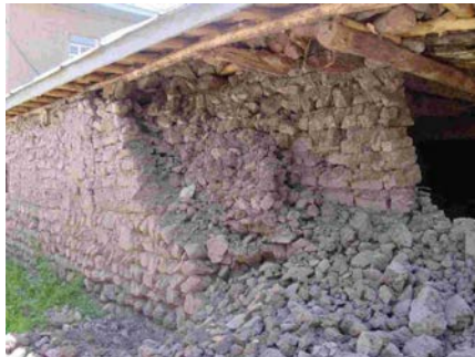
Figure 23a: Typical external walls damage in Firoozabad-Kagoor earthquakes [3]
