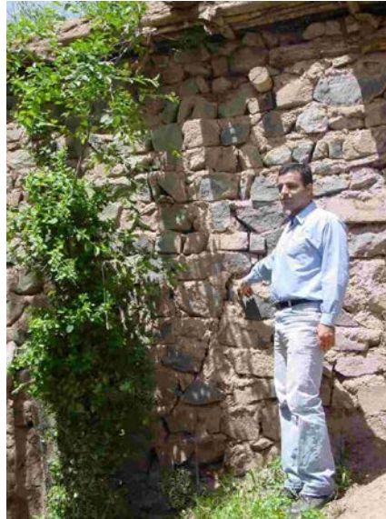
Figure 23b: Typical external walls damage in Firoozabad-Kagoor earthquakes [3]
