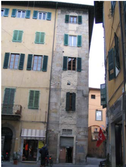
Figure 2: Typical early version of tower: very slender structure with stone pillars.
