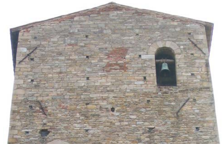
Figure 12: Opposite walls are connected by the use of tie-rods, with evident improvement in seismic behavior.
