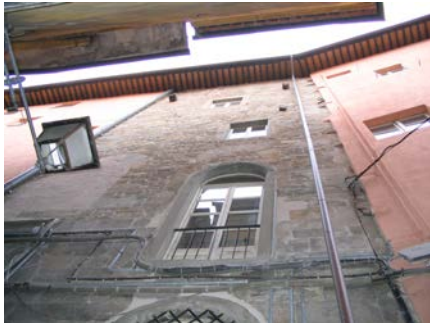
Figure 7: Example of modified position of openings in the facade
