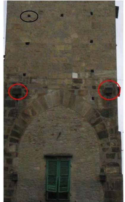
Figure 9: "Il Campano" (bell tower): detail of the holes (black circle) made to support the framework (while the tower was being built) and the balcony after it was finished. The balconies were also strengthened by wood beams supported by shaped stones (r
