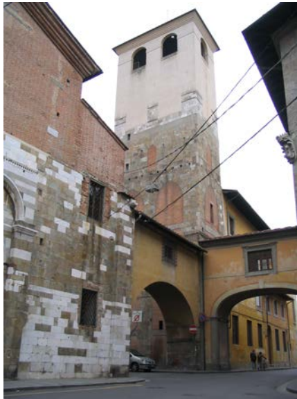
Figure 13: "Torre della Verga d'oro." Structural reinforcements: two large arched openings supporting horizontal forces at the base of the tower have been infilled by clay units.
