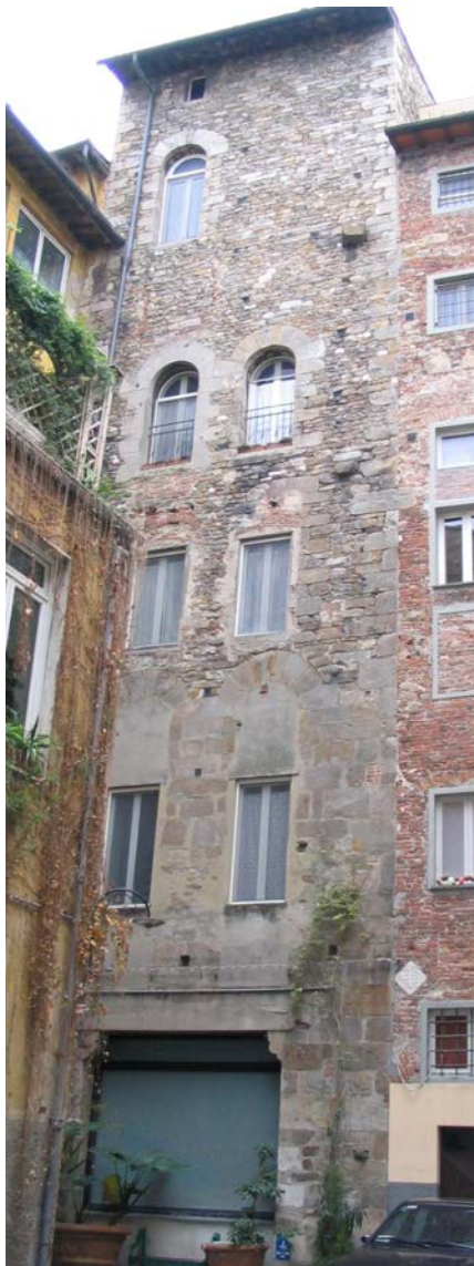
Figure 8: East tower of S. Martino alla Pietra (beginning of 12th century). It has been incorporated into adjacent buildings. Structural deficiencies have been caused by the subsequent unaligned openings as well as by the wide doorways at the ground-floor
