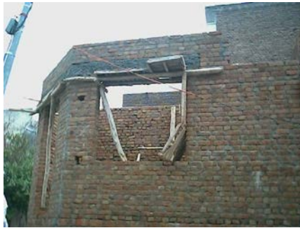
Figure 5: Discontinuity of lintel beams
