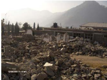
Figure 13: DHQ Garhi Habibullah (NWFP, Pakistan): collapsed buildings constructed with
