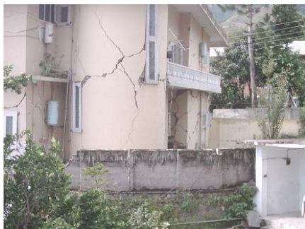
Figure 10: Typical Scissor type cracks in a two story brick masonry house at Muzaffarabad, Kashmir (from Kashmir earthquake Oct 08, 2005)
