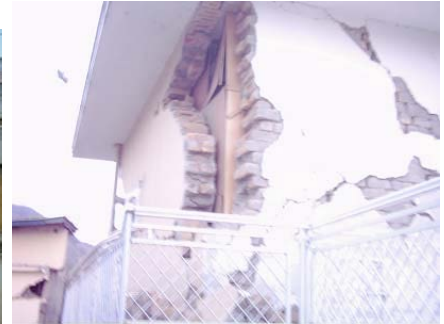
Figure 9: Corner failure in a two story brick masonry house at Muzaffarabad, Kashmir, (from Kashmir earthquake Oct 08, 2005)
