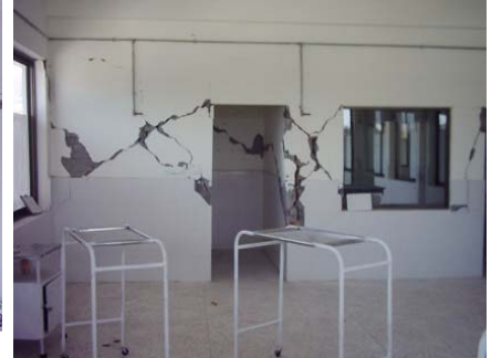
Figure 12: Typical cracks in pier. Manserhra Hospital NWFP Pakistan (from Kashmir earthquake Oct 08, 2005)
