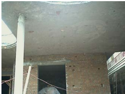
Figure 7: Poor quality of RC work in roof slab (A large number of bricks are placed in RC work to save cement concrete)
