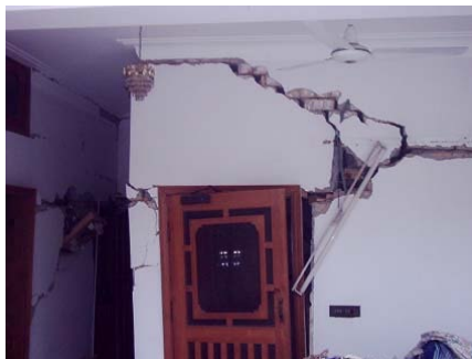
Cracks above door opening and along Figure 11: lintel in a 4.5 inch (125 mm) thick wall in a partition wall in a house at Muzaffarabad, Kashmir, (from Kashmir earthquake Oct 08, 2005)
