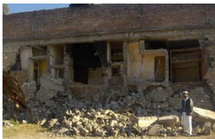
Figure 14: Shinkiarri (NWFP Pakistan): out of plane flexural failure of load bearing wall constructed with block masonry. Note 6ft high
