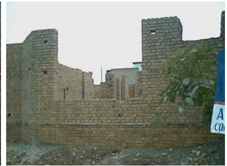
Figure 6: Large openings in walls
