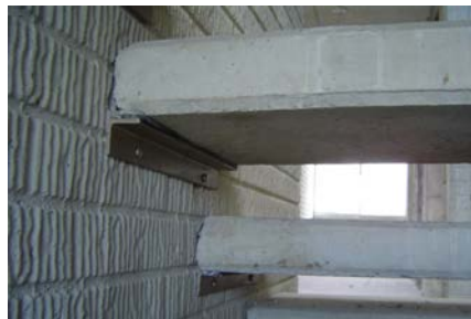
Figure 7. Precast stair supports. OPTIMA S.A. construction project.
