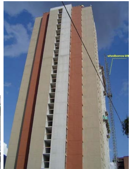
Figure 5c. Wheelbarrow lift structure to transport concrete up to high floors. OPTIMA S.A. construction project.
