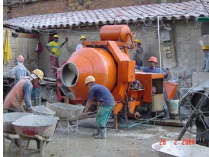
Figure 5b. Workers waiting to fill wheelbarrows from the concrete mixer.
