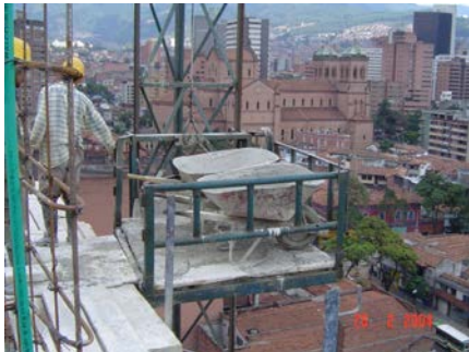
Figure 5d. Wheelbarrow lift stopped at the 19th level. Workers waiting for the wheelbarrows. OPTIMA S.A. construction project.
