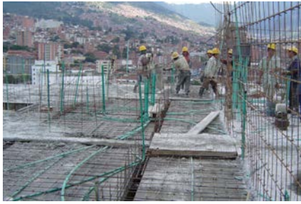
Figure 6c. Concrete placement into walls and slab. Note the preparation of the upper level walls and placement of the electrical nets. OPTIMA S.A. construction project.
