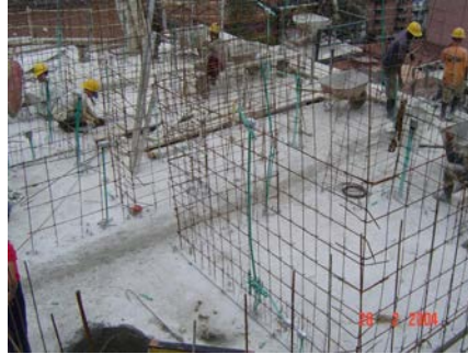
Figure 6d. Wall's reinforcement already placed and armed. OPTIMA S.A. construction project.
