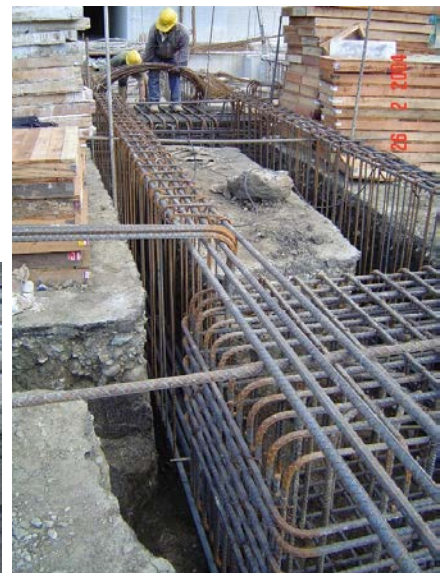
Figure 6b. Perspective view of the reinforcement foundation beams. OPTIMA S.A. construction
