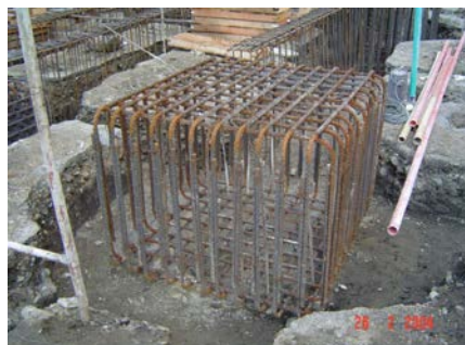
Figure 6a. Cap's reinforcement basket of a hollow
