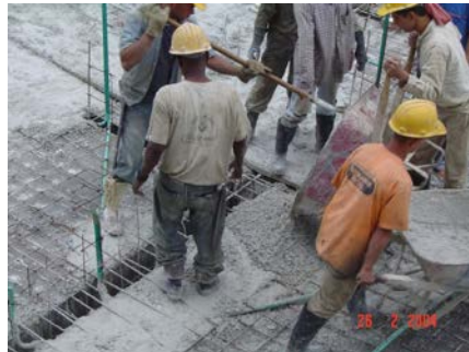
Figure 5e. Concrete placement into the form work. OPTIMA S.A. construction project.
