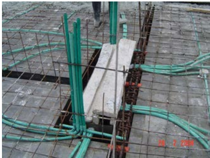
Figure 6f. Opening in the slab for the hydraulics and electrical nets. OPTIMA S.A. construction project.
