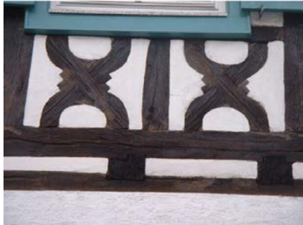
Figure 17: Parapet ornaments: top - at a house in Wildungen, built in the middle till end 16th century. Source: Uhde(1903), Fig. 288 on page 252; bottom - at a house in Durlach. Photo: M. Kauffmann.
