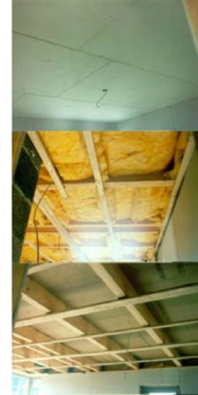
Figure 21: Construction details of floors (new building): from bottom to top different steps in finishing.
