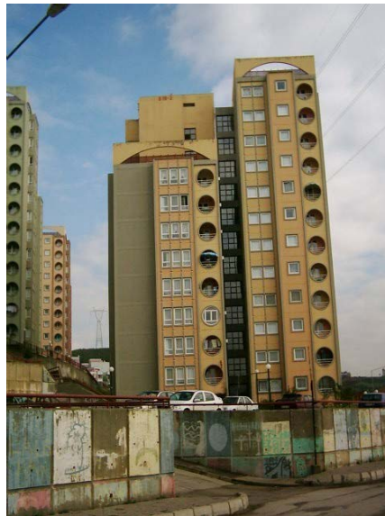
Figure 17: The Post-Earthquake Condition of Another Tunnel Form Building of a Different Housing Complex in İzmit
