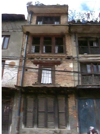
Figure 11: Alteration of original layout. Note vertical division of property, addition of one story and replacement of timber floors with concrete flat slab.
