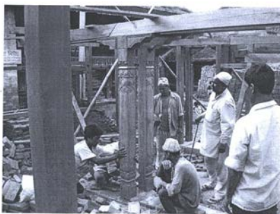
Figure 21: Khokana VDC Office. Detail of positioning of the internal dalan columns. Vertical pins connect the columns to the lower and upper beam. (courtesy of UMEDP)
