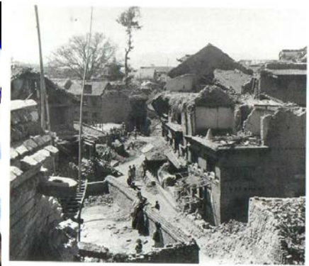
Figure 15: Photograph of a residential street in Lalitpur after the 1934 earthquake.
