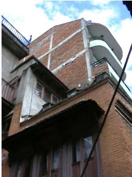
Figure 14: Construction of 5-story concrete frame above a ground floor masonry building
