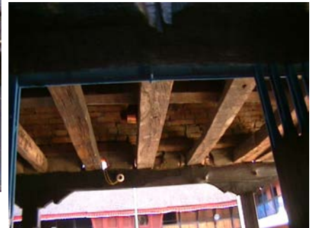
Figure 12: Typical floor structure.
