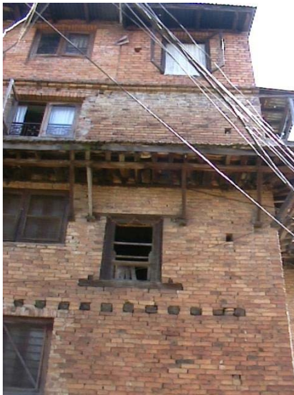
Figure 10: Typical elevation with joists coming through the wall, different window sizes, jetting at third floor level and overhanging of roof. This is sometimes supported by struts.
