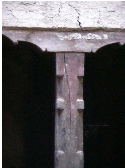
Figure 8: Detail of timber post in the dalan structure.
