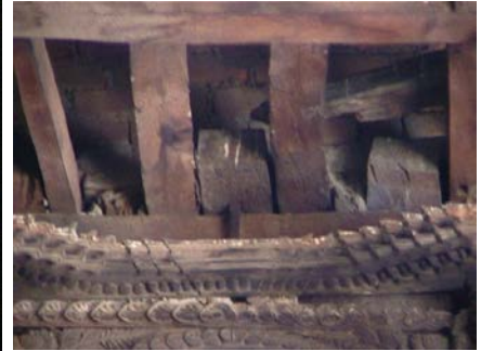
Figure 9: Detail of timber peg connecting joists to walls or transversal beam to limit lateral relative sliding.
