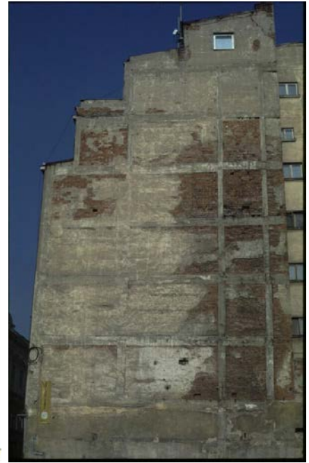
Figure 10: Side wall of a typical building (from Bostenaru(2004))
