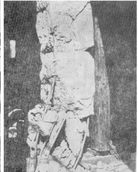
Figure 26: Ground floor column, destroyed due to pounding with neighbouring building (see Balan, 1980: figure VI.20.d. on page 247)
