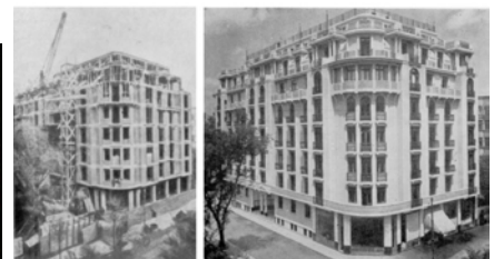
Figure 16: Construction site of a building of similar type (after Prager(1979), Figures 7.4.9. on p. 144 and 7.4.10. on p. 145, featuring on the left the organisation of the building site at block of flats "Spicul" and on the right the finished block)
