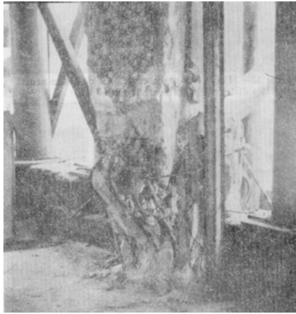
Figure 22: Bending damage at lower node of a column at the same building as image #6 (see Balan, 1980: figure VI.19.a on page 246)
