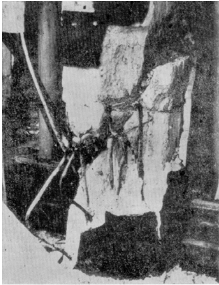
Figure 21: Column destroyed in shear at later demolished building (see Balan, 1980: Figure VI.18.b. on page 246)
