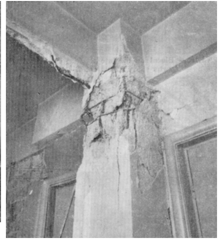
Figure 23: Bending damage at upper end of a column in a block with partial collapse (see Balan, 1980: Figure VI.19:b. on page 246)
