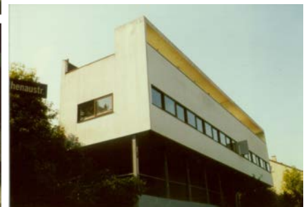
Figure 6: A renewed building of this type: Le Corbusier's building in Stuttgart Weissenhof (from 1927) - a mix of reinforced concrete and metal structure: free standing columns are out of metal.
