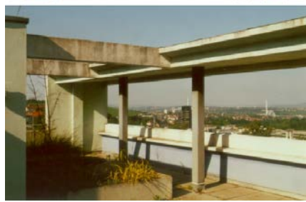
Figure 18: Details showing the way horizontal and vertical (iron) reinforced concrete and vertical metal elements are combined in Le Corbusier's building in Stuttgart Weissenhof.
