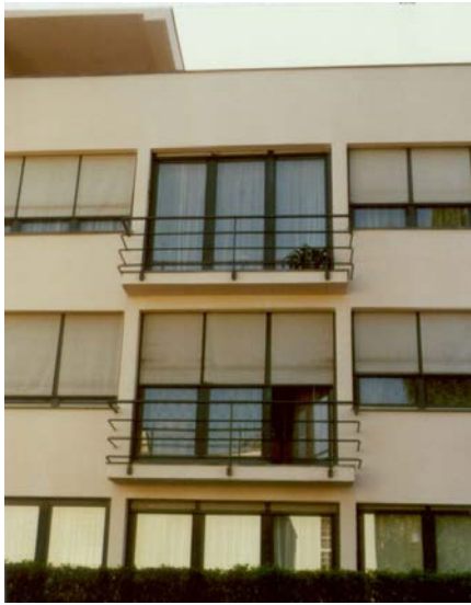
Figure 17: Facade detail from a mid-rise building of this type (Stuttgart).
