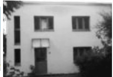
Figure 22: Seismic feature (small openings in infill walls): Facade of a low-rise house (Karlsruhe)
