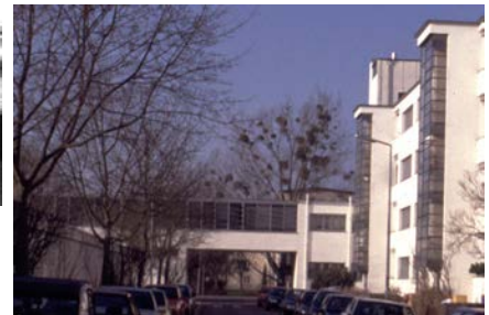
Figure 3: Mid-rise building of this type in context - entry situation in Karlsruhe-Dammerstock
