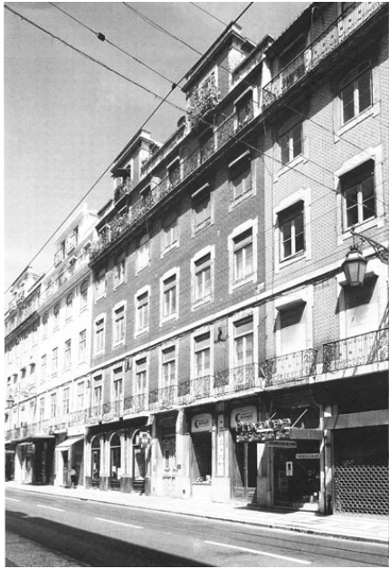
Figure 1: Typical Building (Santos, 2000)
