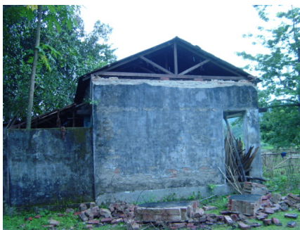
Figure 6: Damage due to 2003 Rangamati Earthquake
