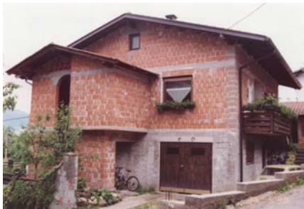
Figure 5C: Key Structural Deficiencies - Missing Bond Beams at the Roof Level and Some Vertical Tie-Columns
