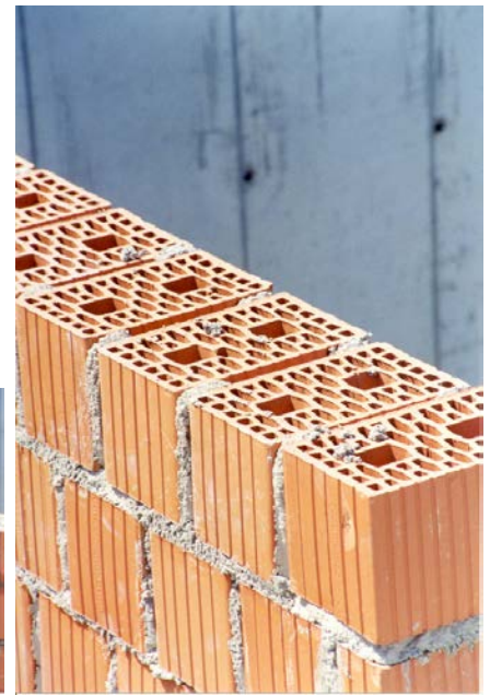
Figure 5B: Key Structural Deficiencies - Head Joints Partially Filled on Both Faces of the Wall
