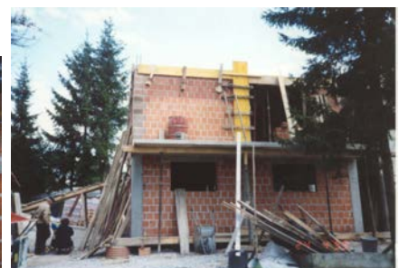
Figure 4C: Critical Structural Details- Reinforced Concrete Tie Columns at the Second Floor Level (note that the columns have been constructed using special blocks with vertical holes)
