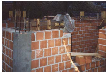
Figure 4B: Critical Structural Details - Reinforced Concrete Tie Columns at the First Floor Level
