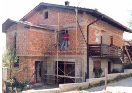
Figure 7: Illustration of Seismic Strengthening Techniques: Construction of the Top Bond Beam (crown beam) in Attics in an existing house
