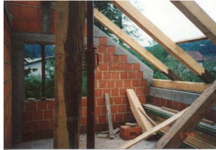
Figure 4E: Critical Structural Details - A Typical Timber Roof and the Bond Beam (crown beam)
