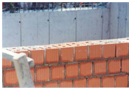
Figure 5A: Key Structural Deficiencies - Masonry Units Absorb the Moisture from the Mortar
