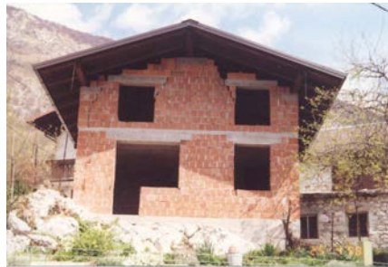
Figure 6: Typical Earthquake Damage: A House without Vertical Tie-Columns and without Top Bond-Beams in Attics (1988 Bovec earthquake)
