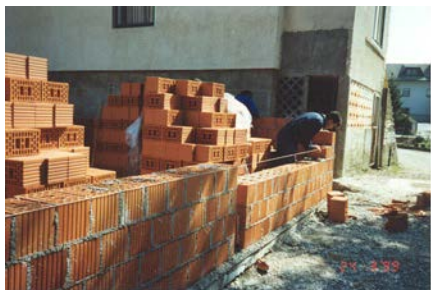
Figure 4A: Critical Structural Details - Masonry Wall Construction
