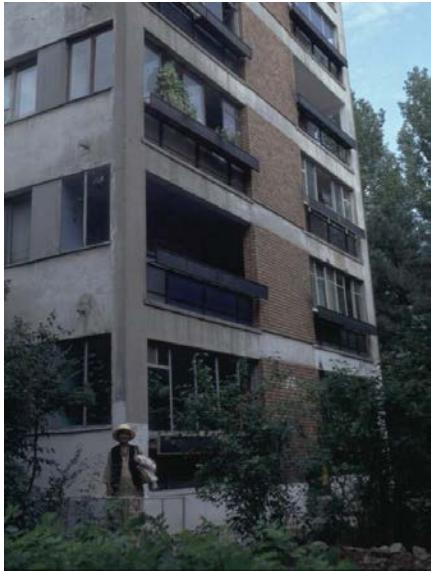
Figure 4: View of the corner of a typical building
