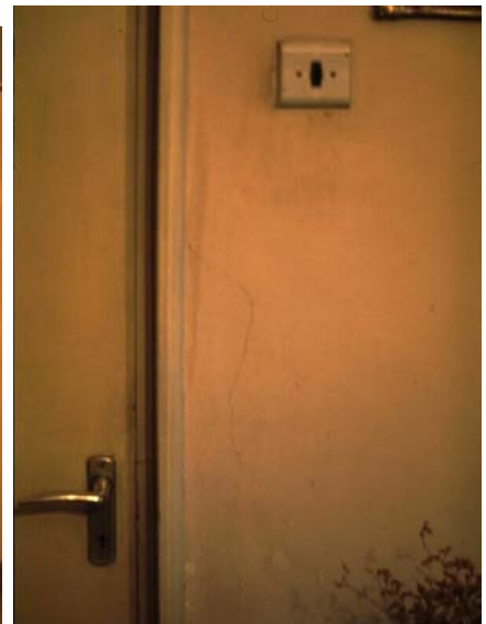
Figure 36: Vertical rift near door.
