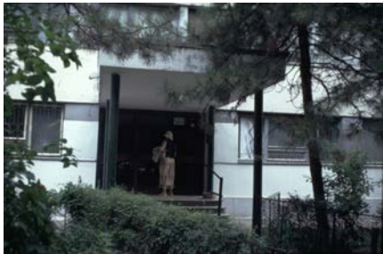
Figure 7: View of the entrance in a typical block.
