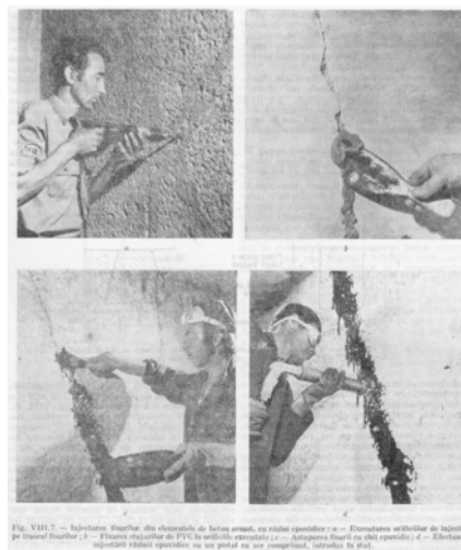
Figure 37: Epoxy resin injections (after Balan, P. 416)
