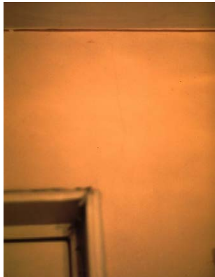
Figure 35: Vertical rift in shear wall going out from door opening corner
