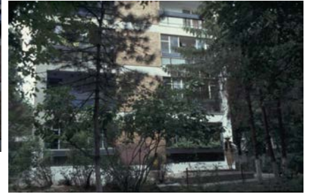
Figure 6: Part of the side view of a typical building.
