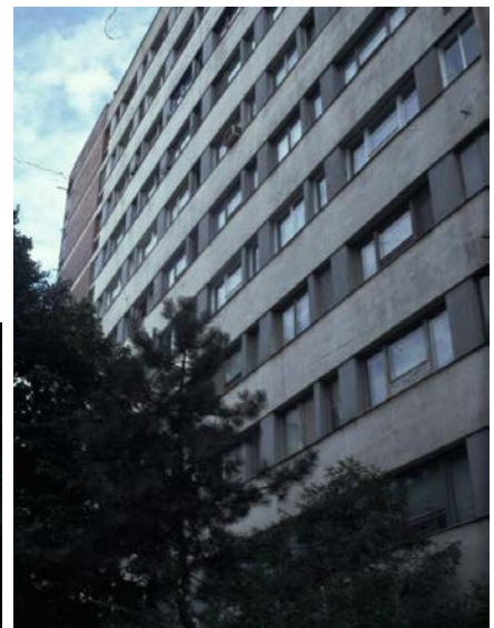
Figure 3: View of the main south facade of a typical building.
