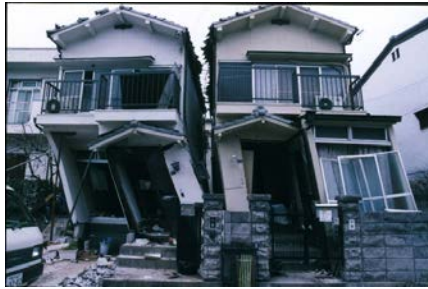
Figure 13: Wooden structure housing damage at the 1995 Kobe earthquake (photo by Michio Miyano)
