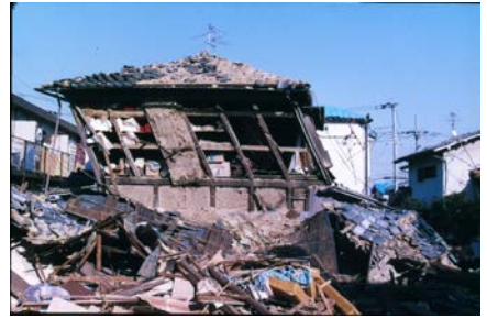
Figure 14: Wooden structure housing damage at the 1995 Kobe earthquake (photo by Michio Miyano)
