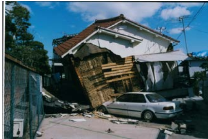
Figure 16: Wooden structure housing damage at the 1995 Kobe earthquake (photo by Michio Miyano)
