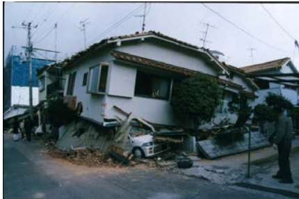
Figure 15: Wooden structure housing damage at the 1995 Kobe earthquake (photo by Michio Miyano)
