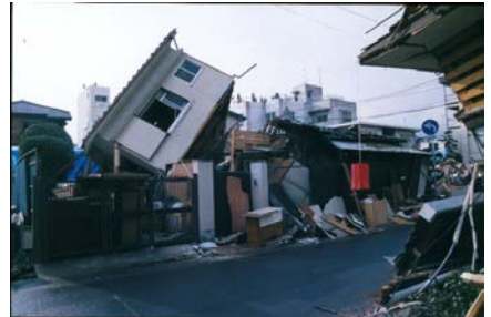
Figure 17: Wooden structure housing damage at the 1995 Kobe earthquake (photo by Michio Miyano)
