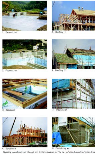
Figure 18: Stages of housing construction (source: http://member.nifty.ne.jp/koso/hokushin/jiban.html )
