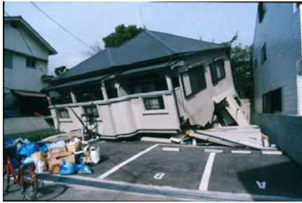
Figure 12: Wooden structure housing damage at the 1995 Kobe earthquake (photo by Michio Miyano)
