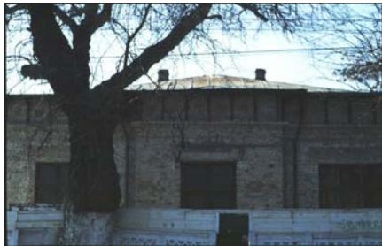
Figure 30: Damage over opening (from Bostenaru, 2004, TAFEL VII)
