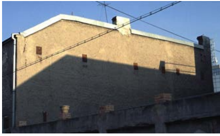
Figure 41: Reinforcement with tension strut, in Romanian "tirant" (from Bostenaru, 2004, TAFEL VII)
