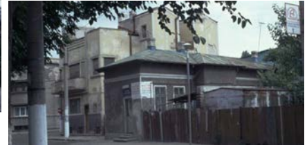
Figure 9: Structural modification: one closed facade window and one changed to door opening.
