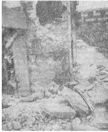
Figure 42: Damages at a vertical post at the corner of a midrise masonry building in the 1977 earthquake. (from Balan, 1980: figure VI.28.b. on page 253)
