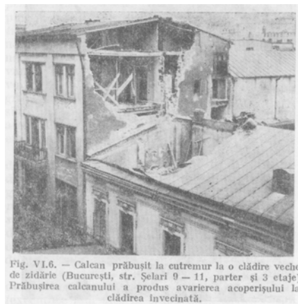
Figure 34: Fallen party wall in neighbouring masonry building, damaging the roof of a building of this type (see Balan, 1980: figure VI.6. on page 234)
