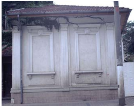
Figure 7: Structural modification: Facade with walled-up windows.
