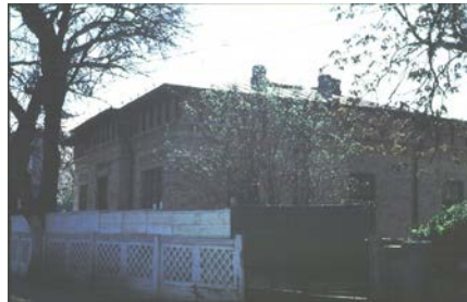
Figure 31: Damage at corner
