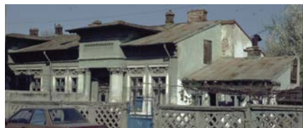
Figure 5: Building from the courtyard side, with added unit over the time (from Bostenaru, 2004, Abb. 2-19 on P. 40)
