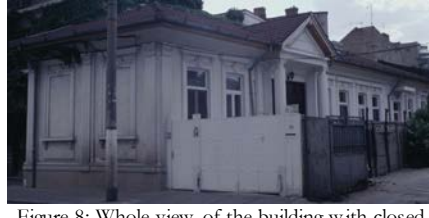
Figure 8: Whole view of the building with closed windows to the street (from Bostenaru, 2004, Abb. 2-4 on P. 24)
