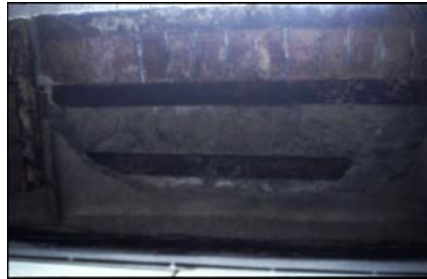
Figure 28: Photo of a brick and metal joists floor structure.
