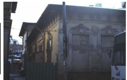
Figure 6: Structural modifications: partial upper floor and closed windows to the street.
