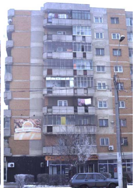
Figure 3: A facade view
