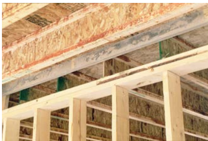
Figure 17: Key seismic deficiency: no blocking between joists at interior load-bearing wall
