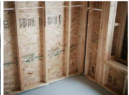
Figure 19: Key seismic deficiency: a typical shear wall without horizontal blocking
