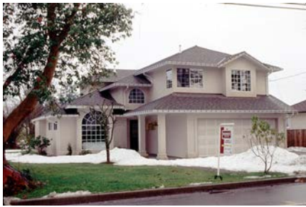
Figure 1: A contemporary two-story wood frame house
