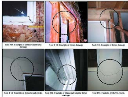
Figure 24: Damage to the two-storey wood frame building specimens tested on the shaking-table: test #13 - 1995 Kobe earthquake, nonengineered building; test 14- 1995 Kobe earthquake, engineered building (Earthquake 99 Project, Source: Kharazzi 2002)
