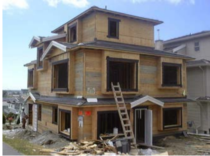
Figure 27: A modern wood frame house under construction (photo courtesy of Dr. G. Taylor)
