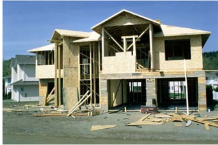
Figure 26: A contemporary two-story wood house under construction
