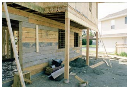
Figure 21: Key seismic deficiency: rear wall of a house - use of horizontal boards
