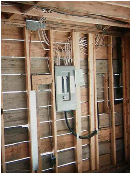
Figure 20: Key seismic deficiency: finger joint and discontinuous studs
