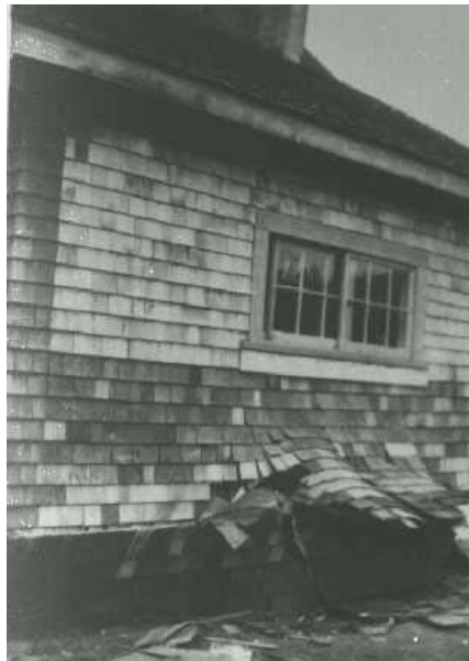
Figure 25: Typical earthquake damage to a wood frame house in Comox, BC in the 1946 earthquake (Source: Natural Resources Canada www.pgc.nrcan.gc.ca/seismo/hist/list.htm )
