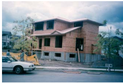
Figure 2: Modern Canadian style single-family woodframe construction with OSB sheathing
