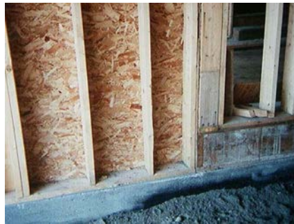
Figure 18: Key seismic deficiency: a typical shear wall without hold-down
