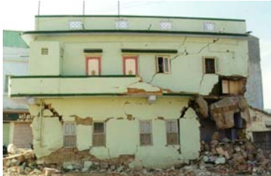
Figure 12: Seismic deficiencies: in-plane shear wall failure (2001 Bhuj earthquake)
