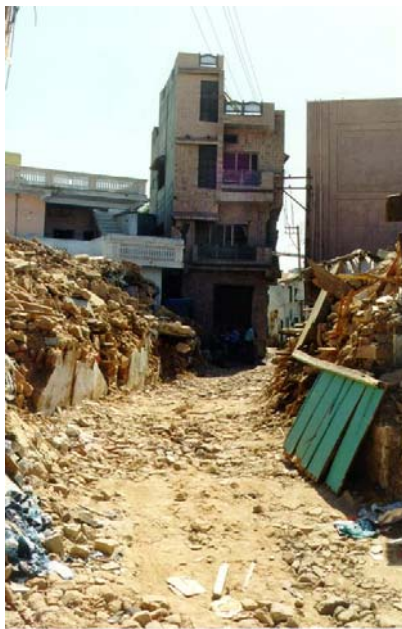
Figure 1: Typical Suburban Building
