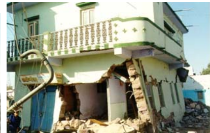
Figure 13: Seismic deficiencies: improper wall-concrete floor slab connection resulting in the out-of-plane wall
