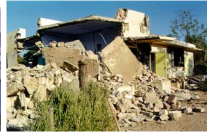
Figure 19: Building Collapse due to the Torsional Motion of Reinforced Concrete (RCC) Roof Slab (2001 Bhuj Earthquake)
