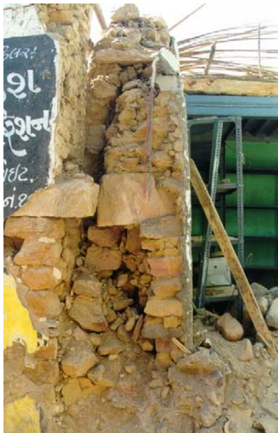
Figure 5: Key details: multi-wythe wall construction
