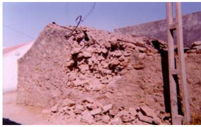
Figure 17: Earthquake damage: out-of-plane wall corner failure (2001 Bhuj Earthquake)
