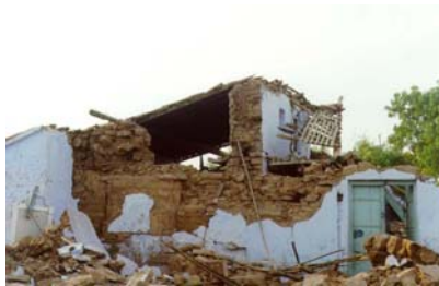
Figure 11: Seismic deficiencies: collapse of stone masonry building due to inadequate wall connections (2001 Bhuj earthquake)
