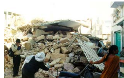
Figure 16: Earthquake damage: complete collapse of a stone masonry building due to inadequate mortar strength (2001 Bhuj Earthquake)
