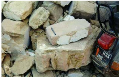
Figure 8: Key details: size of stones used in construction
