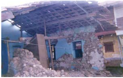
Figure 18: Building Collapse due to Lack of Earthquake Resistant Features (2001 Bhuj Earthquake)
