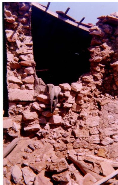
Figure 15: Seismic deficiencies: poor mortar strength in stone masonry walls resulting in the wall collapse (2001 Bhuj Earthquake)
