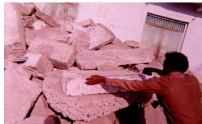
Figure 7: Key details: stone lintels
