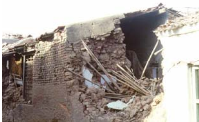
Figure 14: Seismic deficiencies: separation of wall wythes due to absence of through-stones (2001 Bhuj earthquake)
