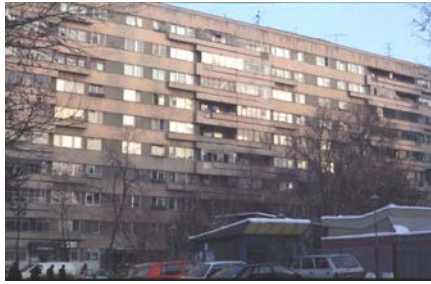
Figure 1A: Typical Building
