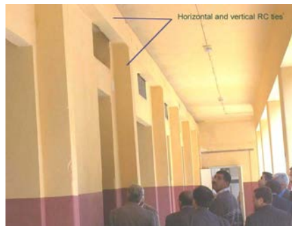
Figure 6B: Seismic Strengthening Techniques: An Example of a Strengthened Building with Vertical and Horizontal RC Ties at the First Floor Level
