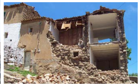
Figure 5F: Totally collapsed stone masonry building in Delys (Boumerdes) in the May 21, 2003 earthquake
