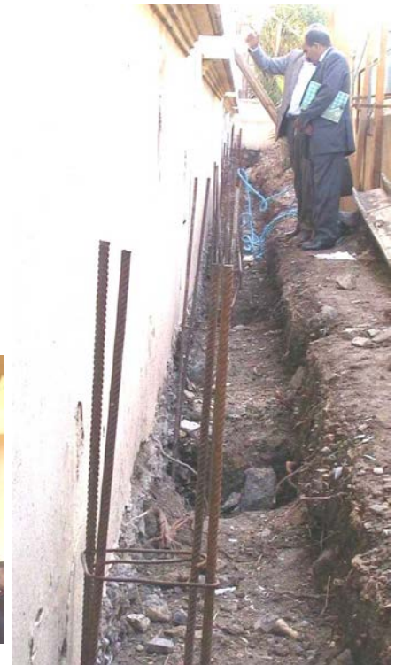
Figure 6C: Seismic Strengthening Techniques: Construction of RC Ties
