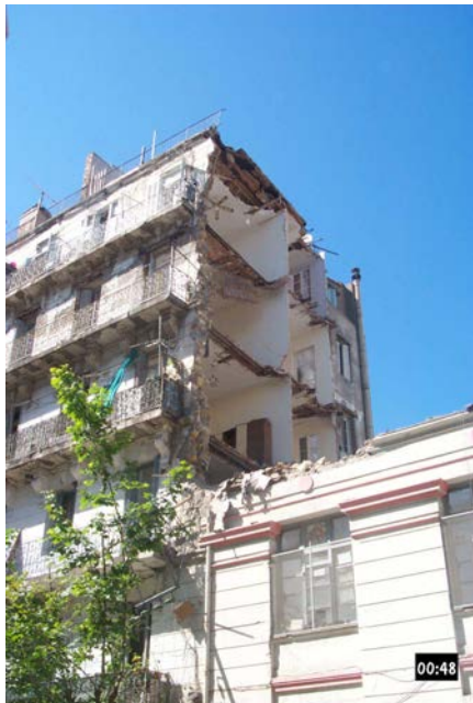
Figure 5D: Damage to a stone masonry building in Algiers in the May 21, 2003 earthquake
