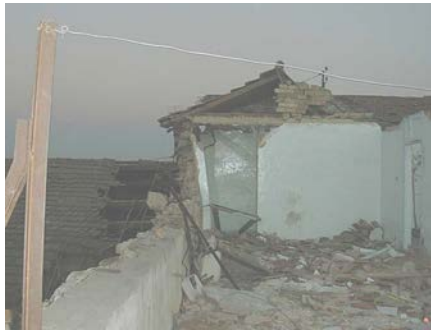
Figure 5A: Typical Earthquake Damage: Partial Roof Collapse (1999 Ain-Temouchent Earthquake)
