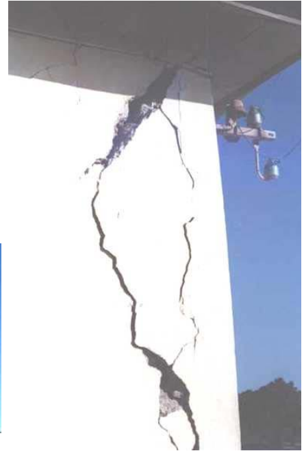
Figure 5C: Typical Earthquake Damage: Cracking in the Wall Corners
