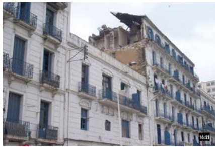
Figure 5E: Collapse of a roof and a side wall in a multi-storey stone masonry building in Algiers city in the May 21, 2003 earthquake
