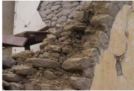
Figure 5I: Collapse of a rubble stone masonry wall made of river stones and mud mortar in the May 21, 2003 earthquake (Sidi Daoud, Boumerdes)
