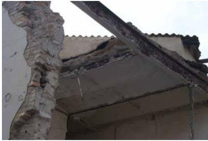
Figure 5G: Collapse of the vaulted brick and steel floor system in the May 21, 2003 earthquake (EI Harrach district, Algiers)
