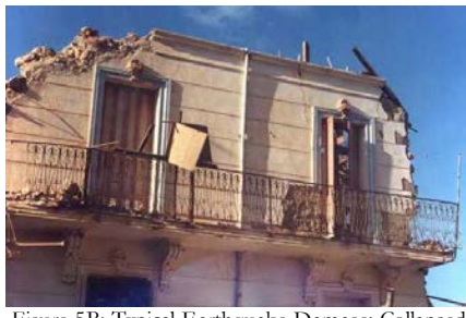
Figure 5B: Typical Earthquake Damage: Collapsed Roof of a Masonry Building (1989 Tipaza Earthquake)
