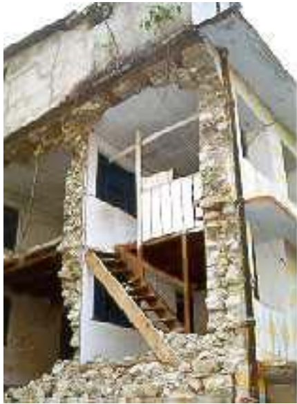
Figure 6D: Typical Earthquake Damage: Out-of-plane Wall Collapse Due to Lack of Anchorage
