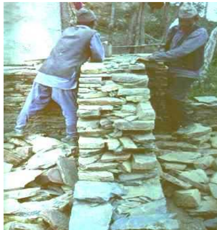
Figure 5: Key Seismic Deficiencies: Lack of Connection Between the Wall Wythes (note loose stone rubble)
