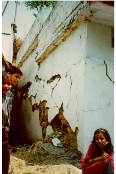
Figure 6E: Typical Earthquake Damage: Wall Bulging Due to Delamination
