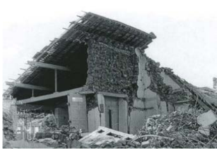
Figure 6A: Typical Earthquake Damage - Delamination of Stone Walls Due to Absence of Bond Stones (through-stones)
