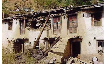
Figure 6B: Typical Earthquake Damage to Stone Masonry Buildings
