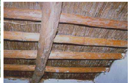
Figure 5A: Seismic Deficiencies: Inadequate Wall-Roof Connections
