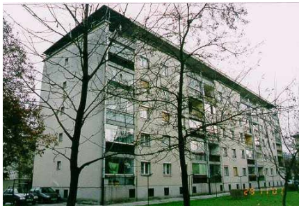
Figure 1A: Typical Building
