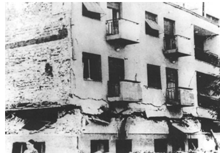
Figure 6B: Typical Earthquake Damage-Severely Damaged Building with Inadequate Wall Density in Predominant Earthquake Direction (1963 Skopje earthquake)
