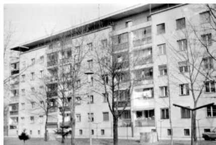
Figure 1B: Typical Building
