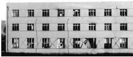
Figure 6A: A Photograph Illustrating Typical Earthquake Damage- Diagonal "X"-type shear cracks in wall piers
