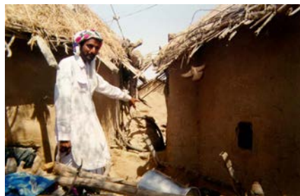
Figure 1A: Typical Building
