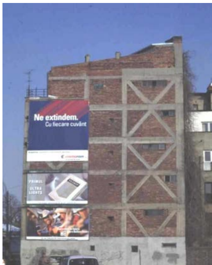
Figure 8A: Another example of a Typical Building (triangular plan, suffered minor damage in the 1977 earthquake)
