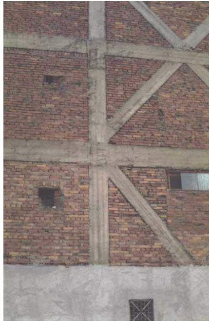
Figure 4B: Critical Structural Details - Frame with Diagonal Bracings and Masonry Infill
