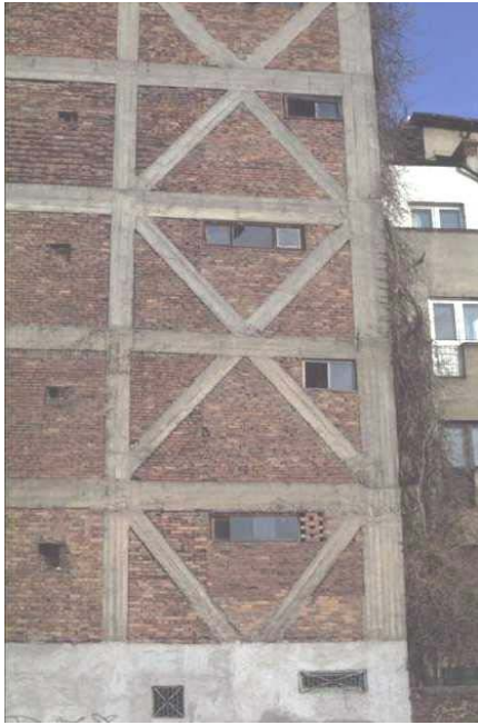
Figure 4A: Critical Structural Details - Frame with Diagonal Braces and Masonry Infill
