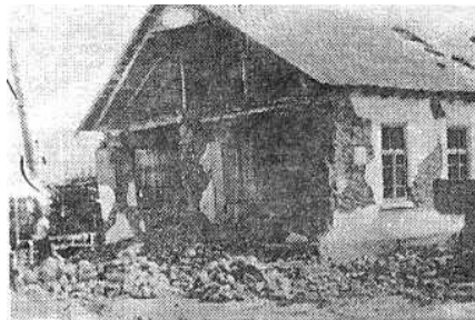
Figure 5: A Photograph Illustrating Typical Earthquake Damage
