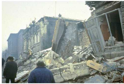
Figure 5: A Photograph Illustrating Typical Earthquake Damage (1988 Armenia earthquake, source: EERI Annotated slide collection)
