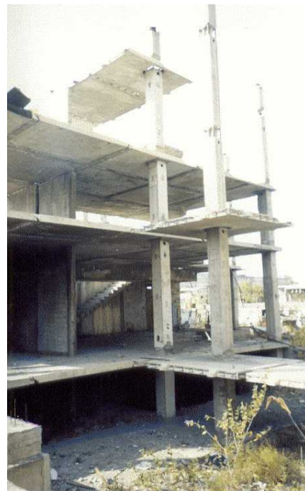
Figure 5: Building under construction
