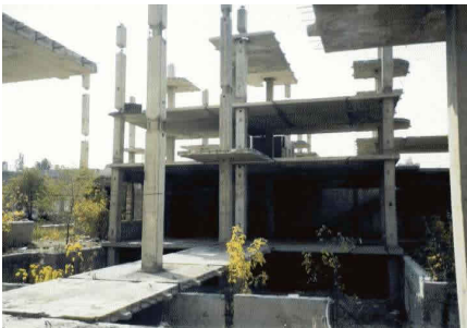
Figure 2A: Key Load-Bearing Elements
