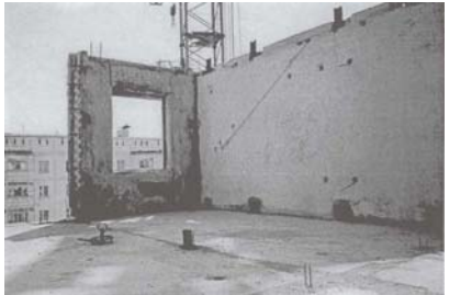
Figure 4H: Building Under Construction, Showing Panel Connections (Source: Imanbekov, Uranova and Iwan, 1999)
