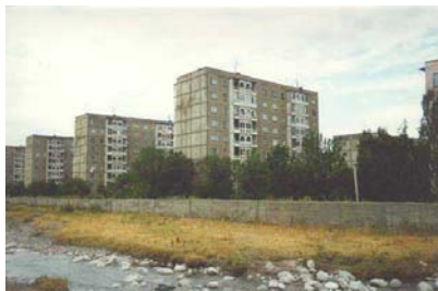
Figure 1A: Typical Building
