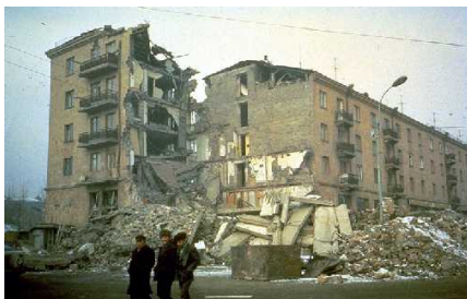
Figure 5A: A Photograph Illustrating Typical Earthquake Damage 1988 Spitak, Armenia earthquake Source: EERI
