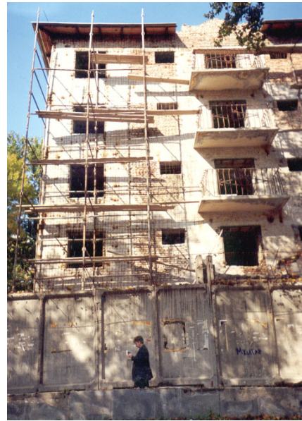
Figure 6B: Seismic strengthening under construction
