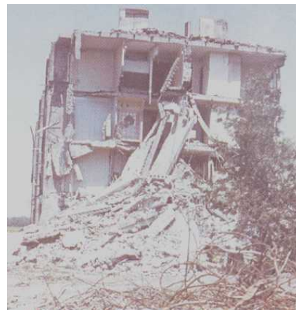
Figure 5B: Building Collapse in the 1988 Spitak, Armenia Earthquake (Source: Klyachko, 1999)
