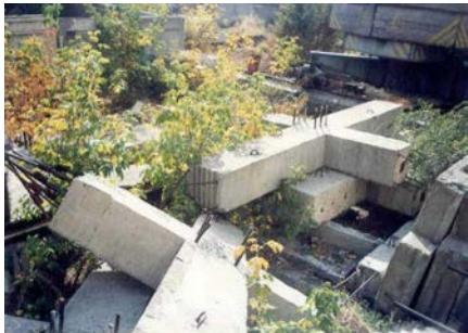
Figure 5: Cruciform Element- as Constructed
