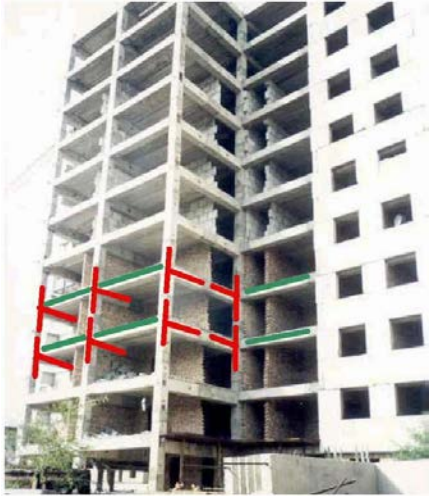
Figure 2A: Key Load-Bearing Elements
