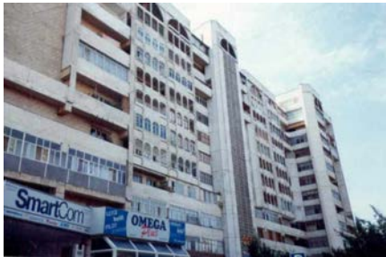
Figure 1A: Typical Building
