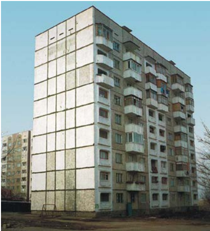
Figure 1A: Typical Building
