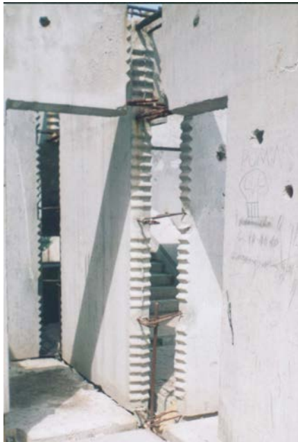
Figure 4E: Critical Structural Details- Serrated Wall Surfaces
