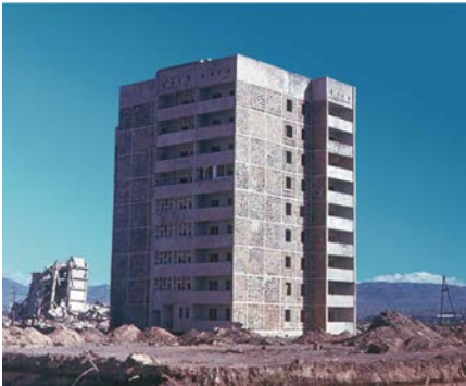
Figure 1B: Typical Building
