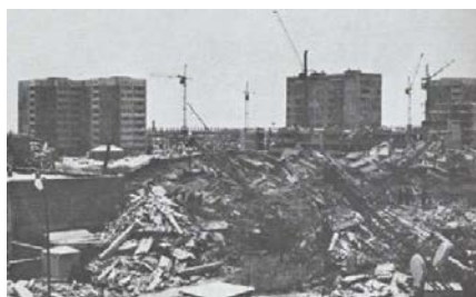
Figure 6: Earthquake Damage - Large Panel Buildings Remained Undamaged in the 1988 Spitak (Armenia) Earthquake (Source: EERI Armenia Earthquake Reconnaissance Report)
