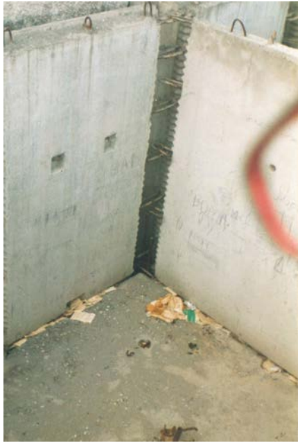
Figure 4B: Critical Structural Details- Vertical Wall Panel Joint
