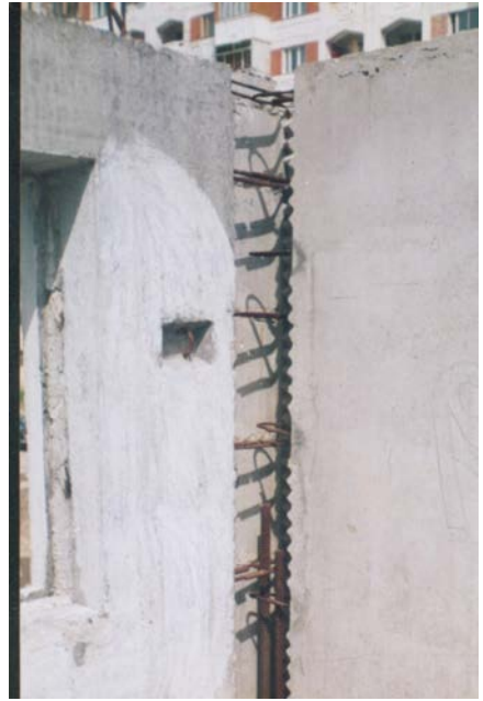
Figure 4C: Critical Structural Details- Vertical Wall Panel Joint
