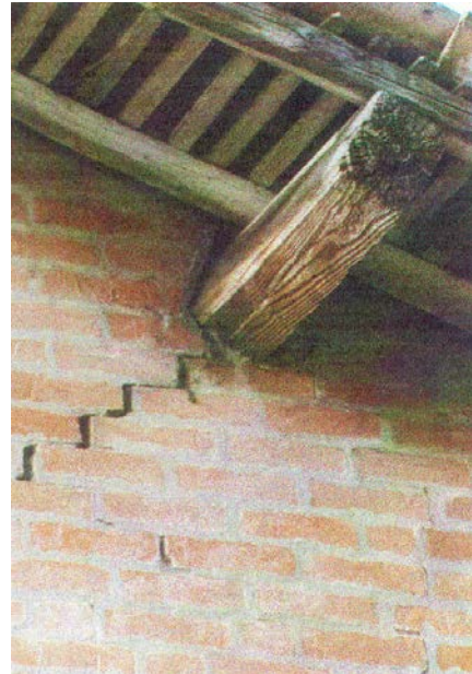
Figure 5B: Wall damage at the roof beam support (1996 Bagnolo earthquake)
