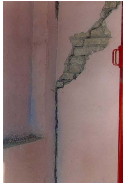
Figure 4: Seismic deficiency- inadequate wall connection
