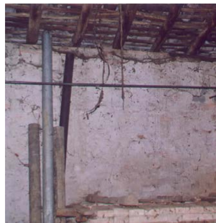
Figure 6B: Seismic strengthening technique - installation of the iron ties
