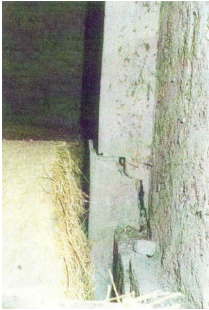
Figure 5A: Wall damage (1996 Bagnolo earthquake)
