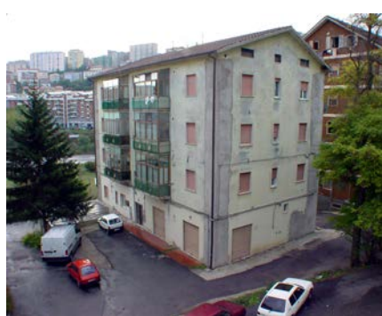
Figure 1B: Typical Building
