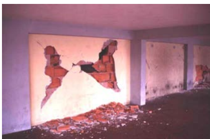
Figure 4A: Typical Earthquake Damage - Cracking of Hollow Clay Tile Partitions
