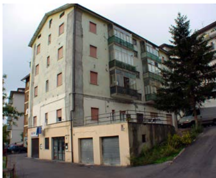
Figure 1A: Typical Building
