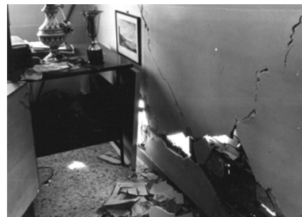
Figure 4B: Typical Earthquake Damage - Cracking of Masonry Partitions
