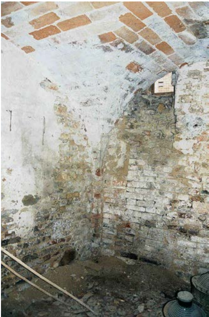
Figure 4B: Brick Walls Supporting the Cross-Vault System
