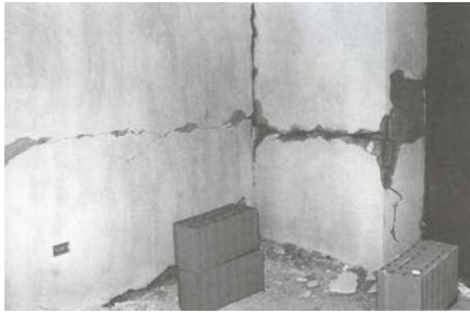
Figure 7G: Seismic Strengthening - Damage of Wall Strengthened by Shotcreting
