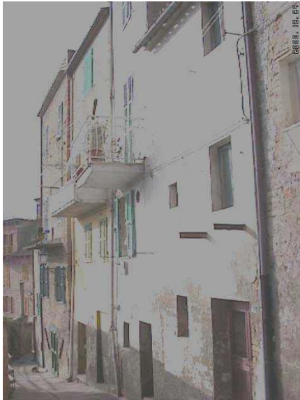
Figure 5A: Key Seismic Deficiencies-Proximity of Windows to the Corners and Vertical Extension of the Building (note also added balconies)
