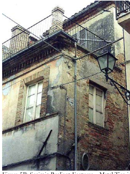
Figure 5B: Seismic-Resilient Features - Metal Ties in two Orthogonal Direction and Brickwork Frame Around Windows
