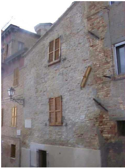
Figure 7A: Illustration of Seismic Strengthening Techniques
