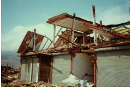
Figure 6A: Building damage in the 1990 Manjil earthquake-collapse caused by the connection failure
