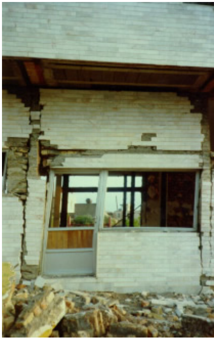
Figure 6D: Failure due to soft story behavior in the 1990 Manjil earthquake
