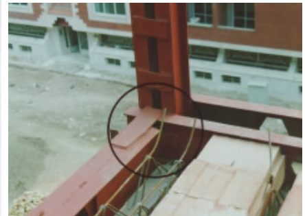
Figure 5A: A seismic deficiency: wrong connection detail
