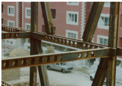
Figure 5B: Seismic deficiency-use of undefined bracing system
