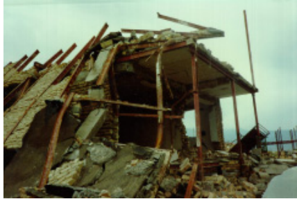
Figure 6B: Building damage in the 1990 Manjil earthquake-collapse caused by the connection failure
