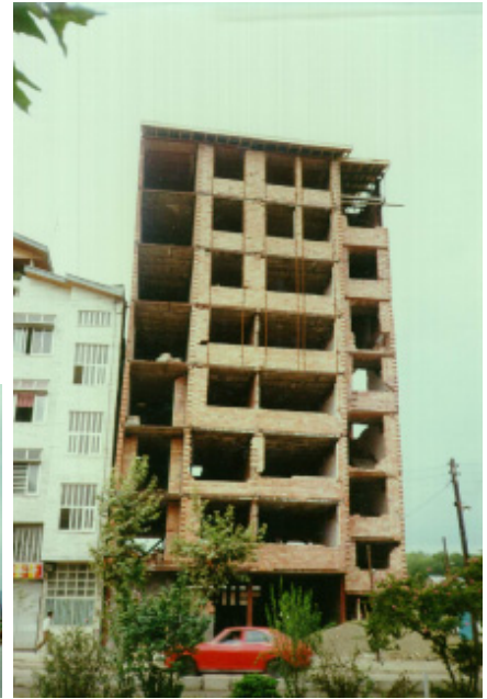
Figure 6C: Minor damage due to pounding between two adjacent buildings in the 1990 Manjil earthquake
