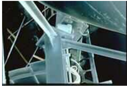
Figure 2C: Typical "Khorjini" connection
