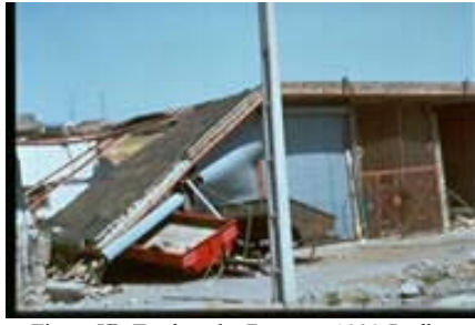
Figure 5B: Earthquake Damage. 1990 Rudbar Manjil Earthquake (EERI Slide Collection)
