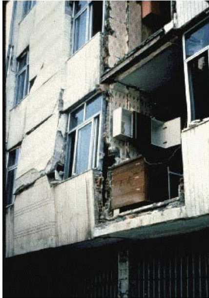
Figure 5E: Earthquake Damage, 1990 Rudbar Manjil Earthquake (EERI Slide Collection)
