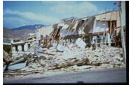
Figure 5C: Earthquake Damage, 1990 Rudbar Manjil Earthquake (EERI Slide Collection)
