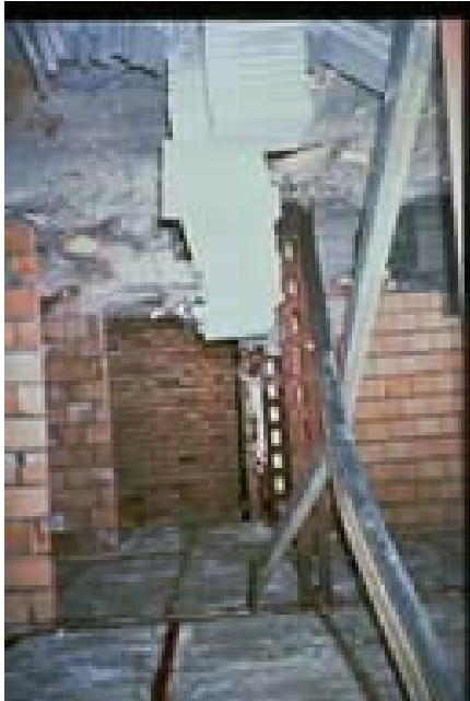
Figure 5D: Earthquake Damage, 1990 Rudbar Manjil Earthquake (EERI Slide Collection)
