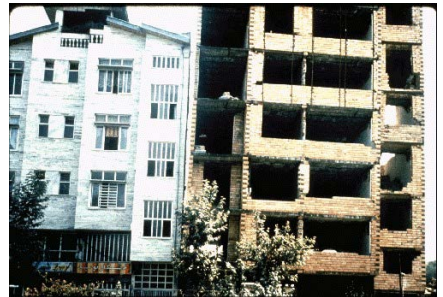
Figure 5F: Earthquake Damage, 1990 Rudbar Manjil Earthquake (EERI Slide Collection)
