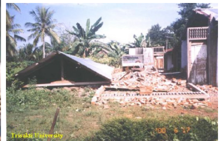
Figure 6C: Unreinforced Brick Masonry Building totally collapsed in the June 4, 2000 Bengkulu Earthquake)
