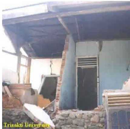
Figure 6B: Typical Earthquake Damage (June 4, 2000 Bengkulu Earthquake)
