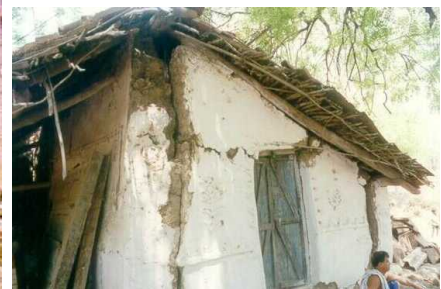
Figure 6A: Typical Earthquake Damage - Cracking and Separation of Walls in the 1997 Jabalpur Earthquake (Source: Sudhir K. Jain, IIT Kanpur)
