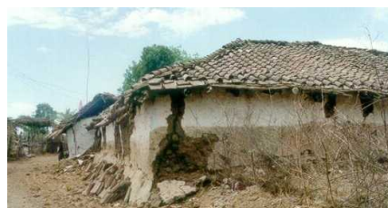
Figure 6C: Typical Earthquake Damage - Cracking and Separation of Walls in the 1997 Jabalpur
