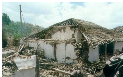
Figure 6B: Typical Earthquake Damage - Collapse of roof in the 1997 Jabalpur Earthquake (Source: BMTPC Publication, 1997, Part-1, Earthen Houses With Clay Tile Roofing Guidelines for Damage Assessment and Post-Earthquake Action)
