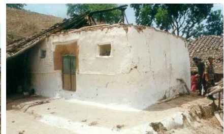
Figure 6D: Typical Earthquake Damage - Cracking of Walls in the 1997 Jabalpur Earthquake (Source: BMTPC Publication, 1997, Part-1, Earthen Houses With Clay Tile Roofing Guidelines for Damage Assessment and Post-Earthquake Action)
