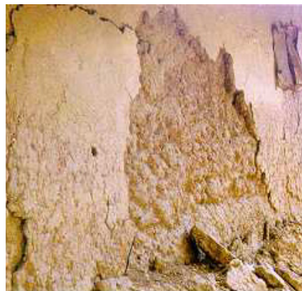
Figure 6: Typical Earthquake Damage
