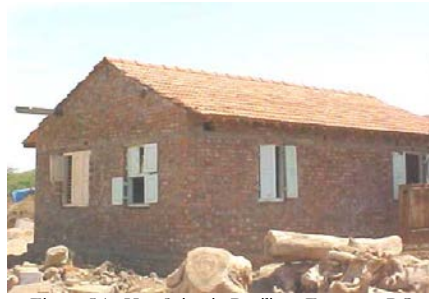
Figure 5A: Key Seismic Resilient Features: RC Lintel Band and Good Quality Brick Masonry Construction (Source: Sudhir K. Jain, IIT Kanpur)
