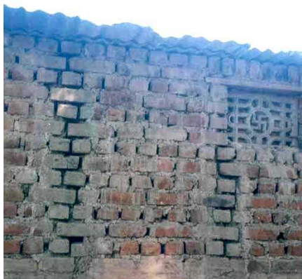
Figure 4: Critical Structural Details: Elevation of Brick Masonry Wall in Mud Mortar (Source: Svetlana Brzev)
