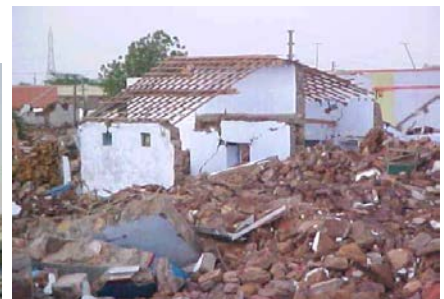
Figure 6C: Typical Earthquake Damage: Collapse of Roof and Walls of a Brick Lime Mortar House in the 2001 Bhuj Earthquake (Source: Sudhir K. Jain, IIT Kanpur)
