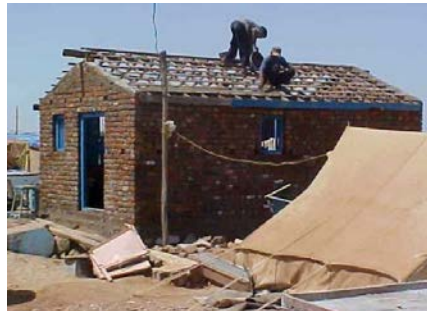
Figure 2B: Key Load-Bearing Elements: Roof Construction (Source: Sudhir K. Jain, IIT Kanpur)
