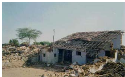
Figure 6B: Failure of a Residential Building, Chobri Village near Bhachau, 2001 Bhuj Earthquake (Source: IIT Powai 2001)
