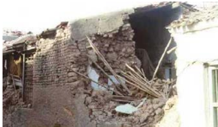
Figure 6A: Typical Earthquake Damage - Wall Collapse Due to Poor Quality Brick Construction and Poor Inadequate Wall Connections in the 2001 Bhuj Earthquake (Source: IIT Powai 2001)
