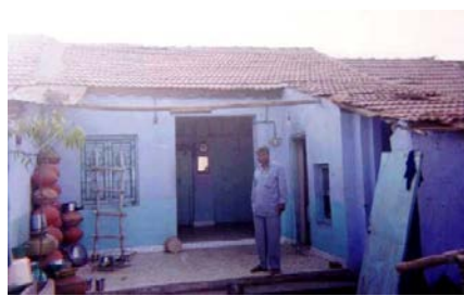
Figure 1A: Typical Rural Building in Maliya Village, Gujarat (Source: IIT Powai 2001)
