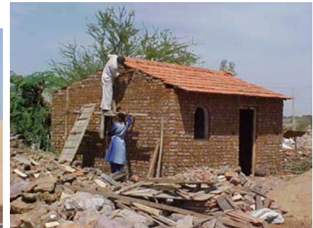
Figure 2C: Key Loadbearing Elements: Laying of Magalore Roof Tiles (Source: Sudhir K. Jain, IIT Kanpur)
