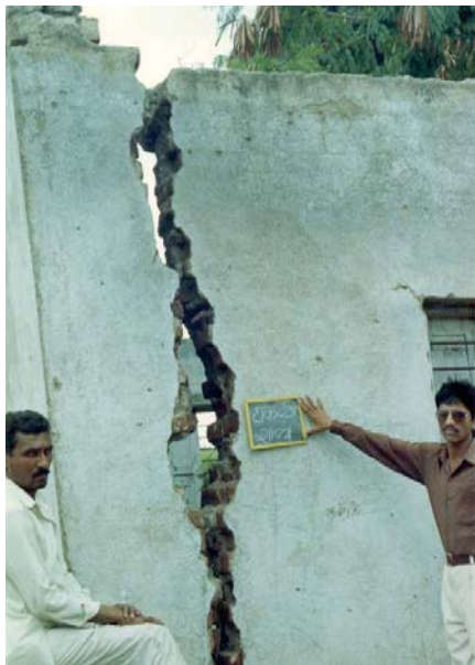
Figure 6D: Typical Earthquake Damage - Wall Corner Failure (1993 Killari Earthquake)
