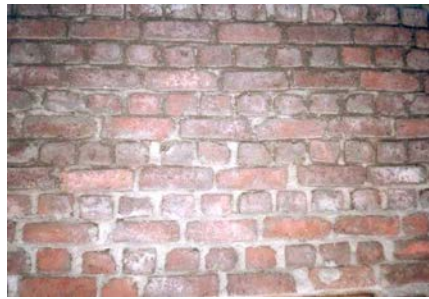
Figure 5B: Construction Deficiency - Excessively Thick Mortar Bedding Joints
