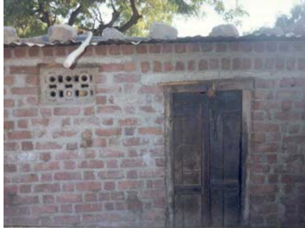
Figure 5D: Construction Deficiency - Discontinuous RC Lintel Band
