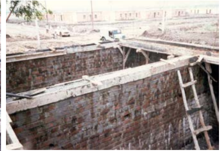
Figure 7F: Construction of RC Lintel Band - Pouring of Concrete Completed
