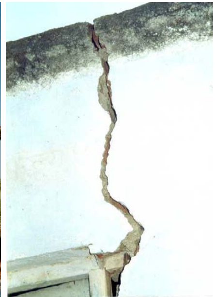
Figure 6C: Typical Earthquake Damage - Wall Cracking above the Door Opening (1993 Killari Earthquake)
