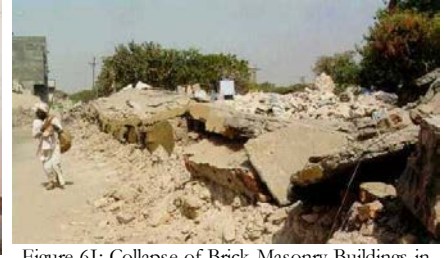
Figure 6I: Collapse of Brick Masonry Buildings in the 2001 Bhuj Earthquake (Source: IIT Pow ai, 2001)
