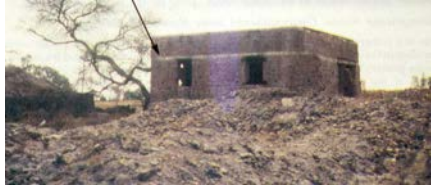
Figure 5A: Key Seismic Resilient Features - RC Lintel Band and Good Quality Construction; note example of a building that sustained the effects of the 1993 Killari earthquake (M6.4) without damage although located very close to the epicentre
