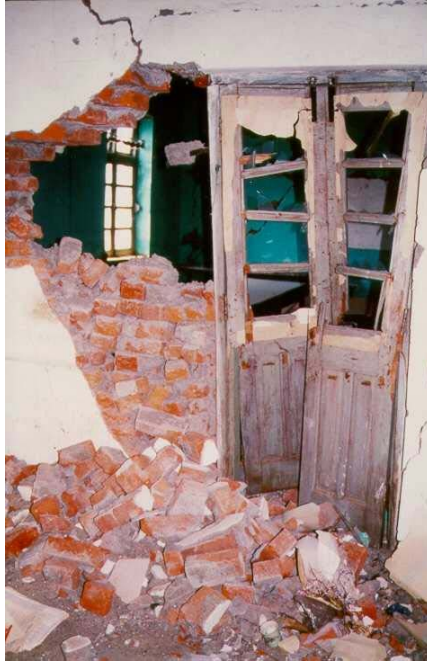
Figure 6H: Failure of Brick Masonry Walls in the 1997 Jabalpur Earthquake
