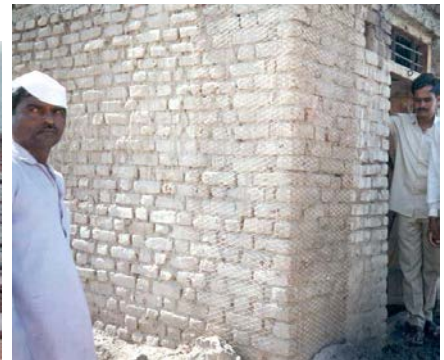
Figure 7C: Seismic Strengthening Techniques - Corner Strengthening
