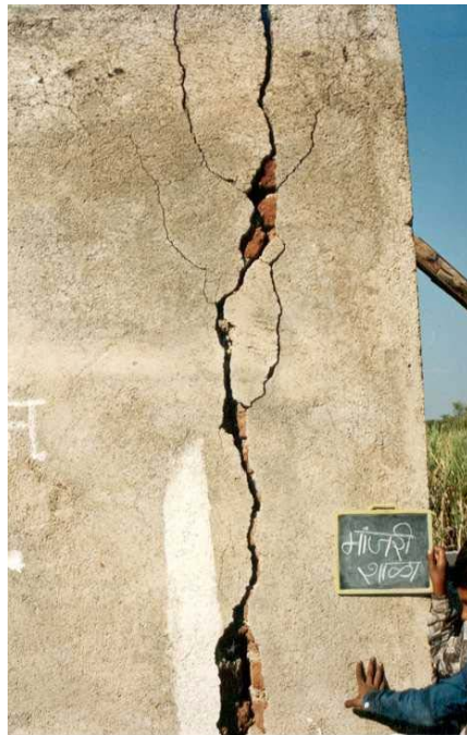
Figure 6B: Typical Earthquake Damage - Wall Corner Cracking (1993 Killari Earthquake)
