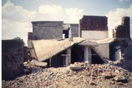
Figure 6A: Typical Earthquake Damage - Roof Collapse Caused by the Wall Collapse (1993 Killari Earthquake)
