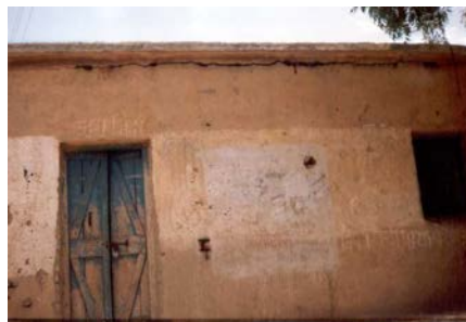
Figure 6E: Typical Earthquake Damage - Sliding Failure of Roof-Wall Connection Due to the Absence of Wall Reinforcement (1993 Killari Earthquake)
