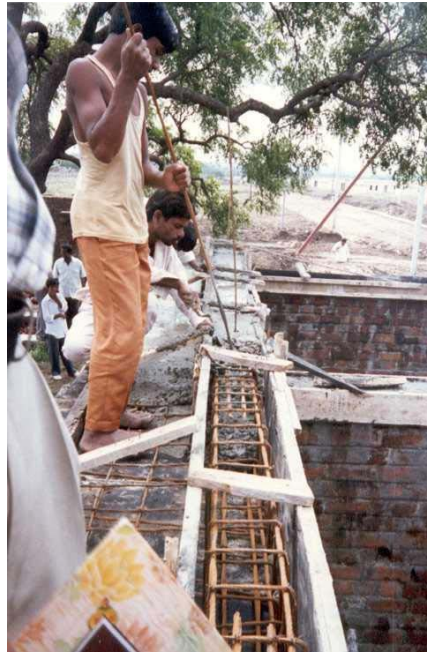
Figure 7E: Construction of RC Lintel Band
