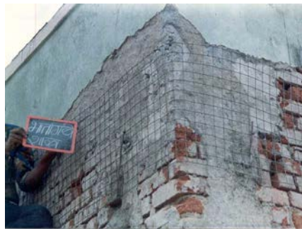
Figure 7B: Seismic Strengthening Techniques - Lintel Bandage
