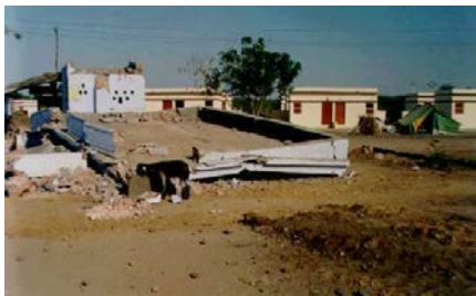
Figure 6J: View of a Collapsed traditional brick masonry building in cement mortar (foreground) and masonry building with lintel bands which sustained only a moderate damage in the 2001 Bhuj earthquake (Source: IIT Pow ai, 2001)
