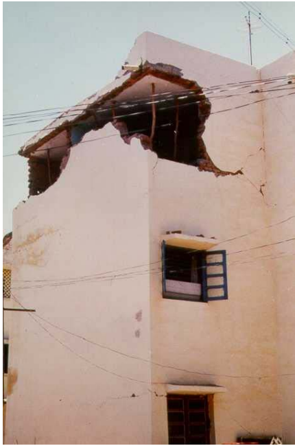
Figure 6G: Partial Building Collapse in the 1997 Jabalpur Earthquake
