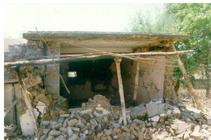
Figure 6B: Typical Earthquake Damage - Failure of Masonry Walls in the 1997 Jabalpur Earthquake (Source: Sudhir K. Jain, IIT Kanpur)
