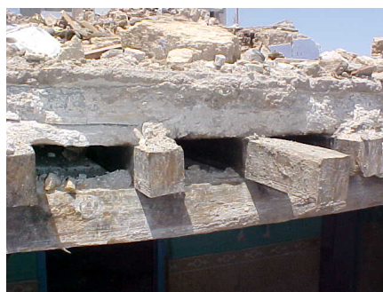
Figure 5: Key Seismic Deficiencies - Heavy Roof
