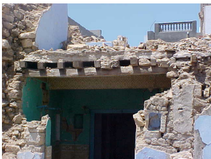
Figure 6: Typical Earthquake Damage in the 2001 Bhuj Earthquake Damage in the 2001 earthquake (Source: Sudhir K. Jain, IIT Kanpur)
