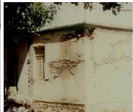
Figure 4B: Critical Structural Details - Unreinforced Brick Masonry Wall in Mud Mortar (1993 Killari Earthquake), Source: Sudhir K. Jain, IIT Kanpur
