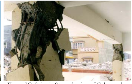
Figure 7C: Seismic Strengthening of Columns by Jacketing from Floor Level - Improper Technique (2001 Bhuj Earthquake)
