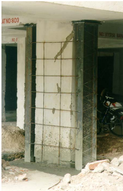
Figure 6G: View of the Intact Portion of an Apartment Building (2001 Bhuj Earthquake)
