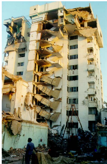
Figure 6H: Failure of Lower Two Stories of the Right Wing of an Apartment Building With Soft Story. Note that the Left Wing Without Soft Story is Apparently Undamaged (2001 Bhuj Earthquake)
