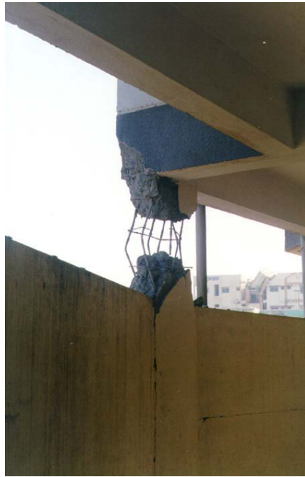
Figure 6B: Improper Reinforcement Detailing of Beam-Column Joint
