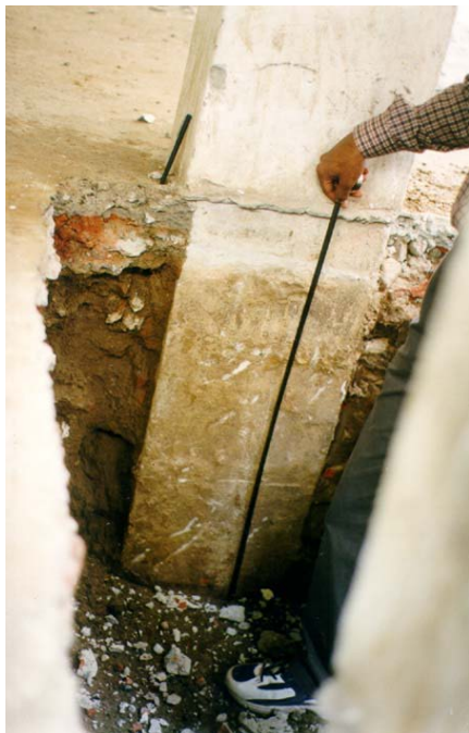
Figure 6A: A Photograph Illustrating Typical Earthquake Damage
