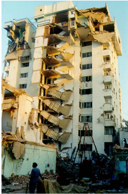
Figure 6A: A Photograph Illustrating Typical Earthquake Damage
