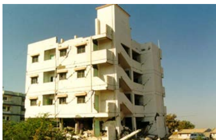
Figure 6J: Shear Failure of Column Just Below the Beam-Column Junction Due to Poor Construction Material and Insufficient Lateral Reinforcement (2001 Bhuj Earthquake)
