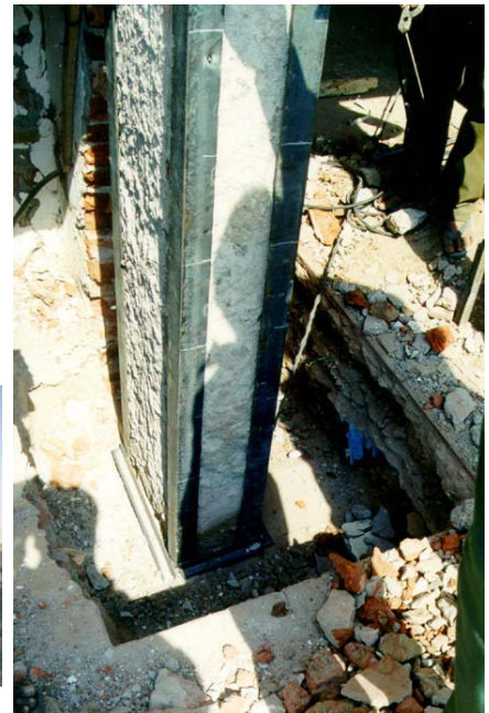
Figure 6F: Failure of Column Below the Beam-Column Joint Due to Short Column Effect
