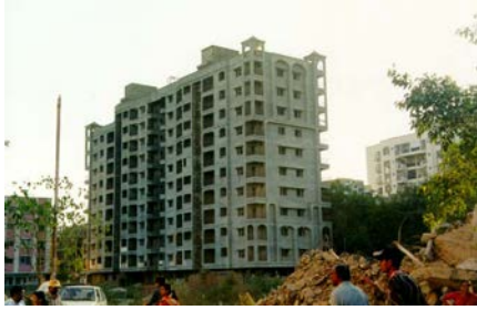
Figure 7D: Termination of Column Jacket Steel at Beam Soffit Level Resulting in No Increase in Moment Capacity of Column (2001 Bhuj Earthquake)
