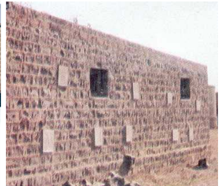
Figure 7H: Seismic Strengthening - An Example of a Retrofitted Building (note through-stones and RC lintel band)
