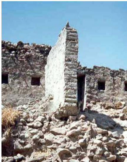
Figure 5C: Structural Deficiency - Absence of Foundations
