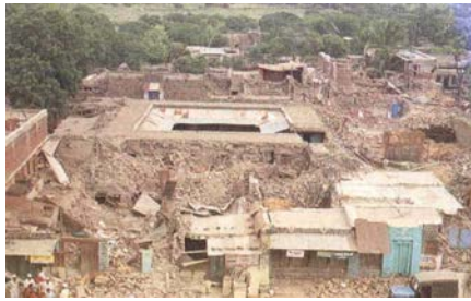
Figure 6: An Areal View of the Killari Village Devastated by the 1993 Earthquake (Source: GSI 1996)
