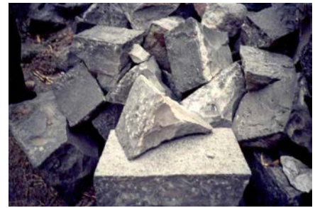
Figure 4E: A Typical Wedged-Shape Stone Used for the Exterior Wall Wythe
