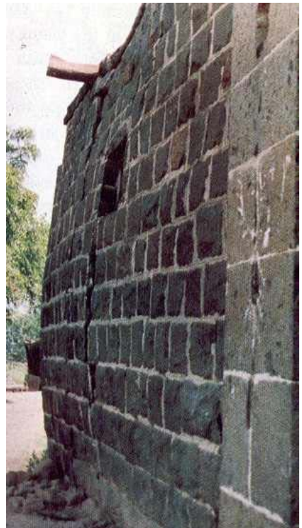
Figure 6E: Typical Earthquake Damage - Building and Cracking of a Thick Stone Wall in the 1993 Killari Earthquake (Source: GSI 1996)
