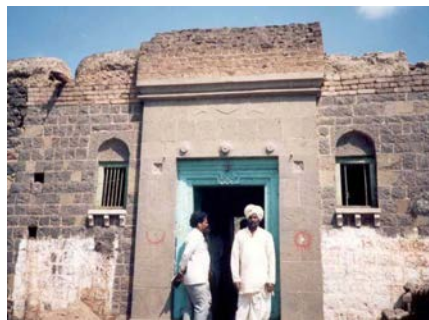
Figure 1A: Typical Building
