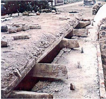
Figure 7C: Seismic Strengthening - Installation of a Bandage at the Lintel Level (an alternative to the installation of RC band) Source: GOM 1998
