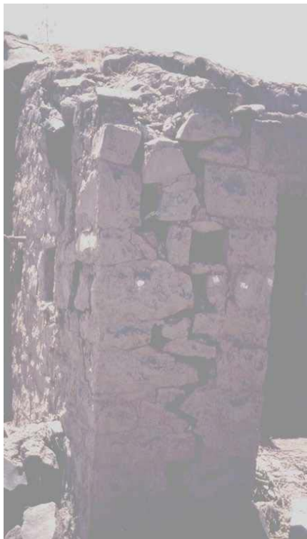
Figure 6D: Typical Earthquake Damage - Delamination of Stone Wall Wythes due to the Absence of Through Stones (1993 Killari earthquake)
