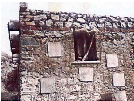
Figure 7I: Seismic Strengthening - An Illustration of Corner Strengthening Technique (Source: GOM 1998)
