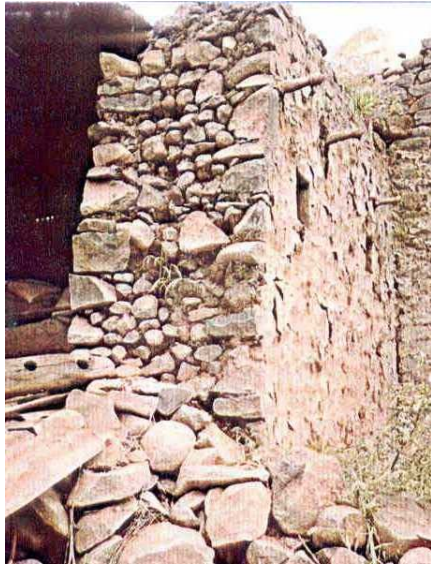
Figure 5: Key Seismic Deficiency - Extremely Thick Stone Walls
