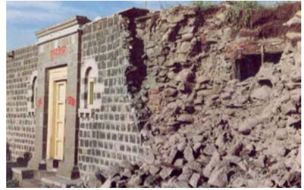
Figure 6B: Typical Earthquake Damage - Partial Collapse of the Exterior Wall in the 1993 Killari earthquake (Salegaon Village, Source: GSI 1996)
