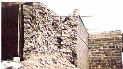
Figure 6C: Typical Earthquake Damage - Delamination of the Exterior Wall Wythe (the interior wythe remained undamaged due to restraint provided by timber posts), 1993 Killari Earthquake
