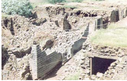
Figure 6A: Massive Collapse of Stone Masonry Buildings in the 1993 Killari Earthquake (Yelvat Village, Source: GSI 1996)
