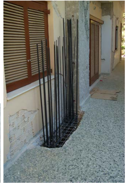
Figure 6C: Seismic Strengthening - Extension of te New Shear Wall Through the Floor Slab
