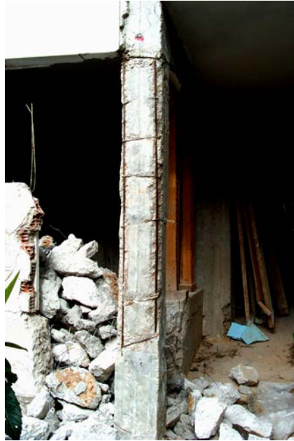
Figure 5: Typical Earthquake Damage to a Column of the Older 1960 Astructure (1999 Athens Earthquake)
