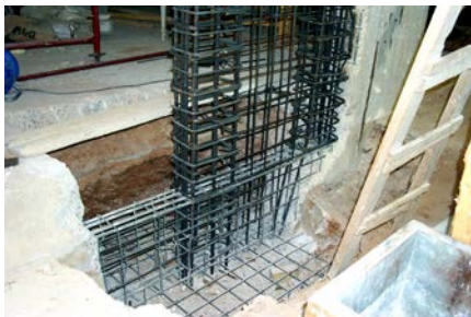
Figure 6D: Seismic Strengthening of the Footing
