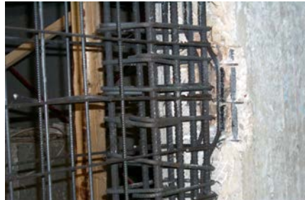
Figure 6B: Seismic Strengthening - Connection of the Old and New Concrete (Welding of Rebars)
