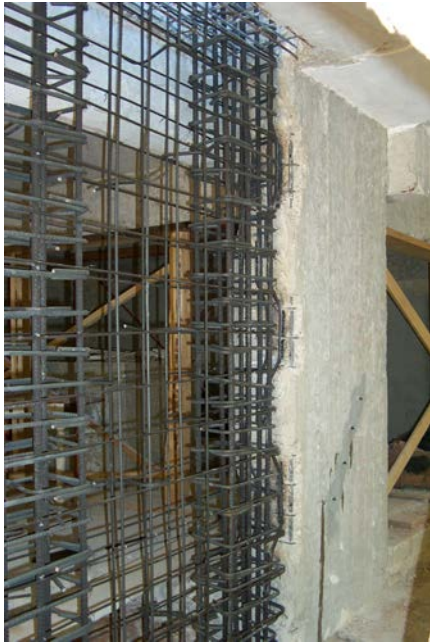
Figure 6A: Seismic-strengthening Techniques - Installation of a New Shear Wall
