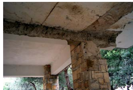
Figure 4: Critical Structural Elements: Column-Floor Slab Connection (1980 Structure)
