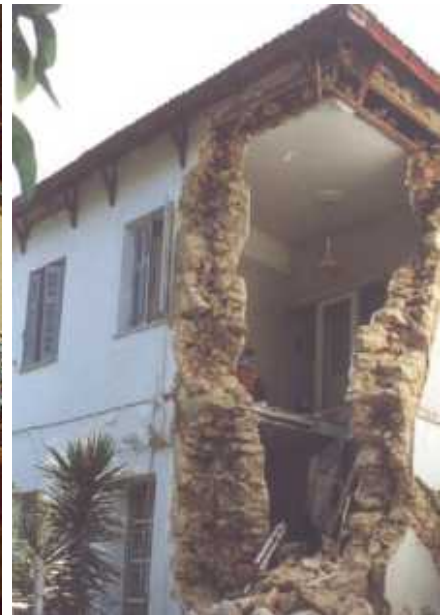
Figure 5C: Partial Collapse of a Stone Masonry House in Nea Philadelphia (1999 Athens earthquake); Source: EERI
