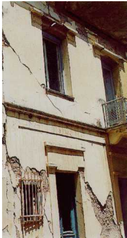
Figure 5B: Typical Earthquake Damage - Falling of Plaster and Shear Cracking of the Walls (1999 Athens Earthquake)
