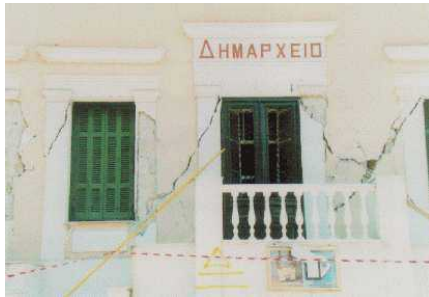
Figure 5A: Typical Earthquake Damage - Shear Cracking of Masonry Walls (1999 Athens earthquake)
