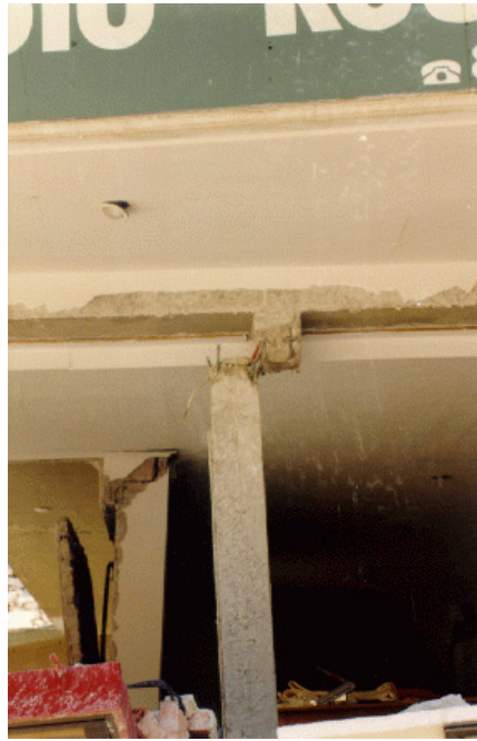
Figure 5B: Building Collapse in the 1999 Athens earthquake
