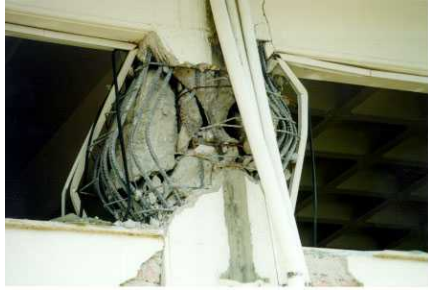
Figure 5D: Typical Earthquake Damage-Column Failure (1999 Athens Earthquake)
