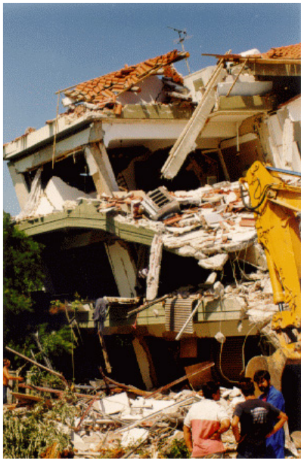
Figure 5A: Typical Earthquake Damage (1999 Athens earthquake)
