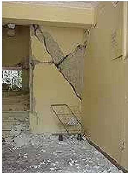
Figure 5E: Failure of column, due to short column effect, of a 5-story building in Ano Liosia, which was built in 1997 according to the new Greek Seismic Code (1999 Athen earthquake); Source: ITSAK
